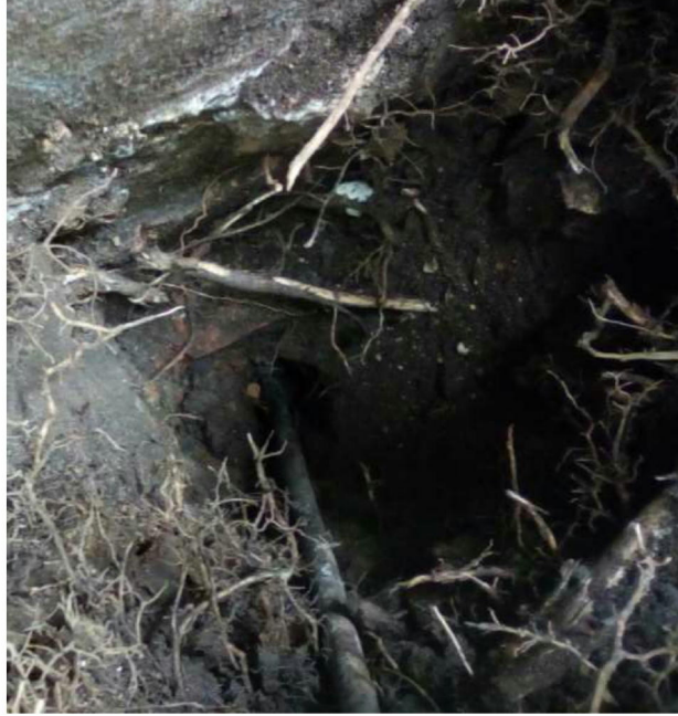
Photo 1 – EH1 Foundation Pit
