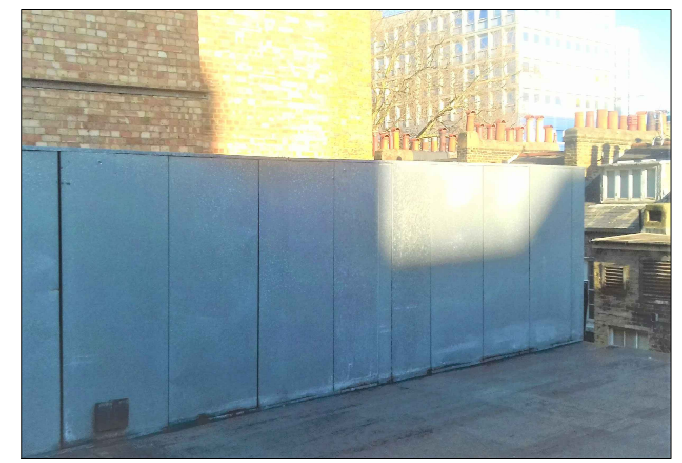
Existing plant screen
