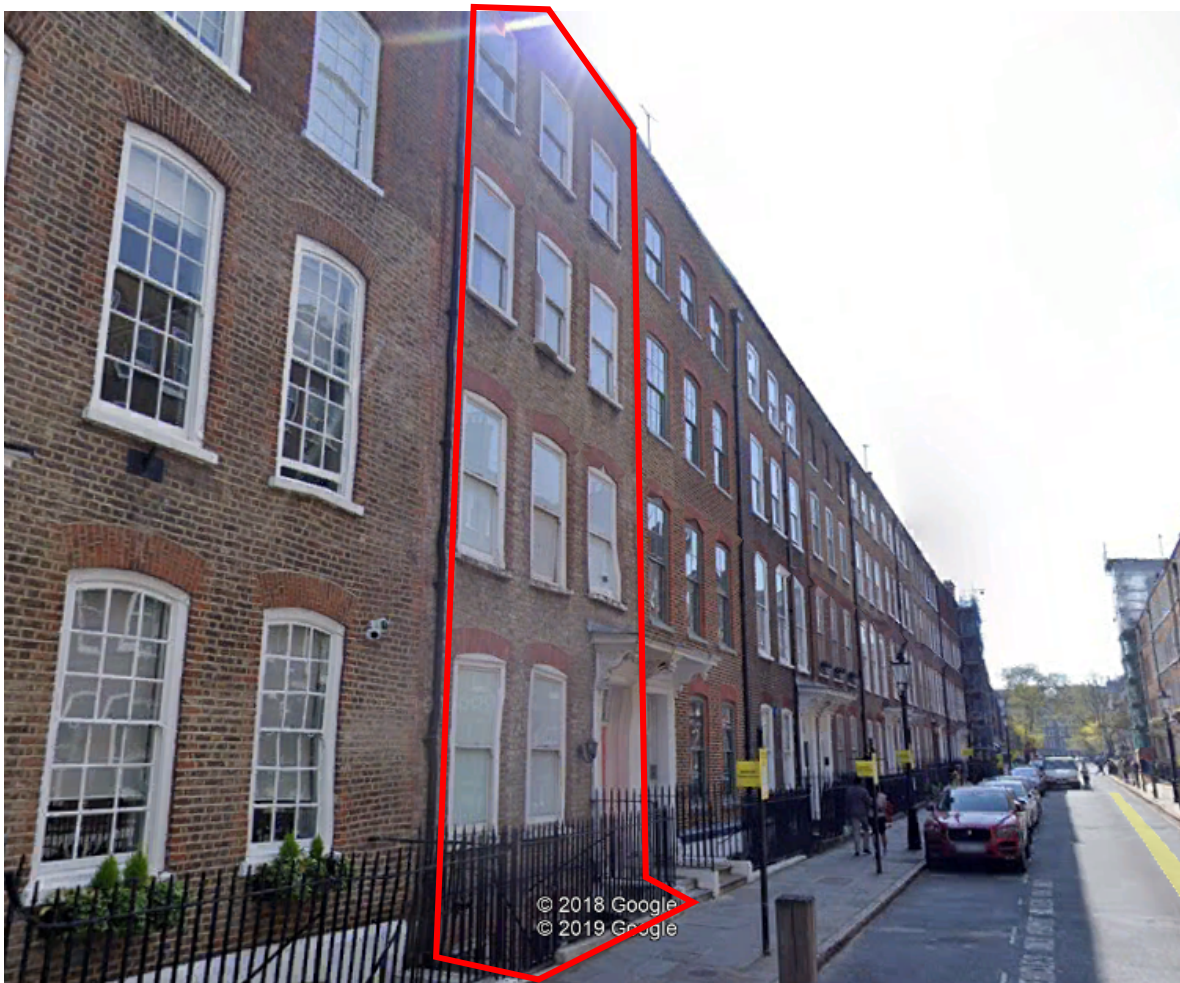
Figure 2: Existing site development at 15 Great James Street. (image courtesy of Google Earth).
