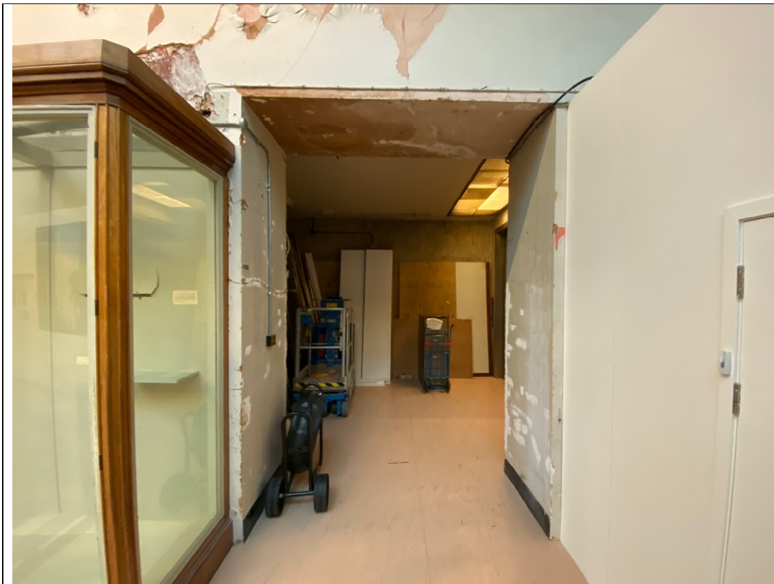
Figure 1: view from Gallery 60 looking south to goods lift lobby
