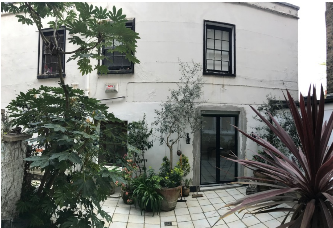
Photo of Front Elevation of Field Cottage showing modified as-built openings
