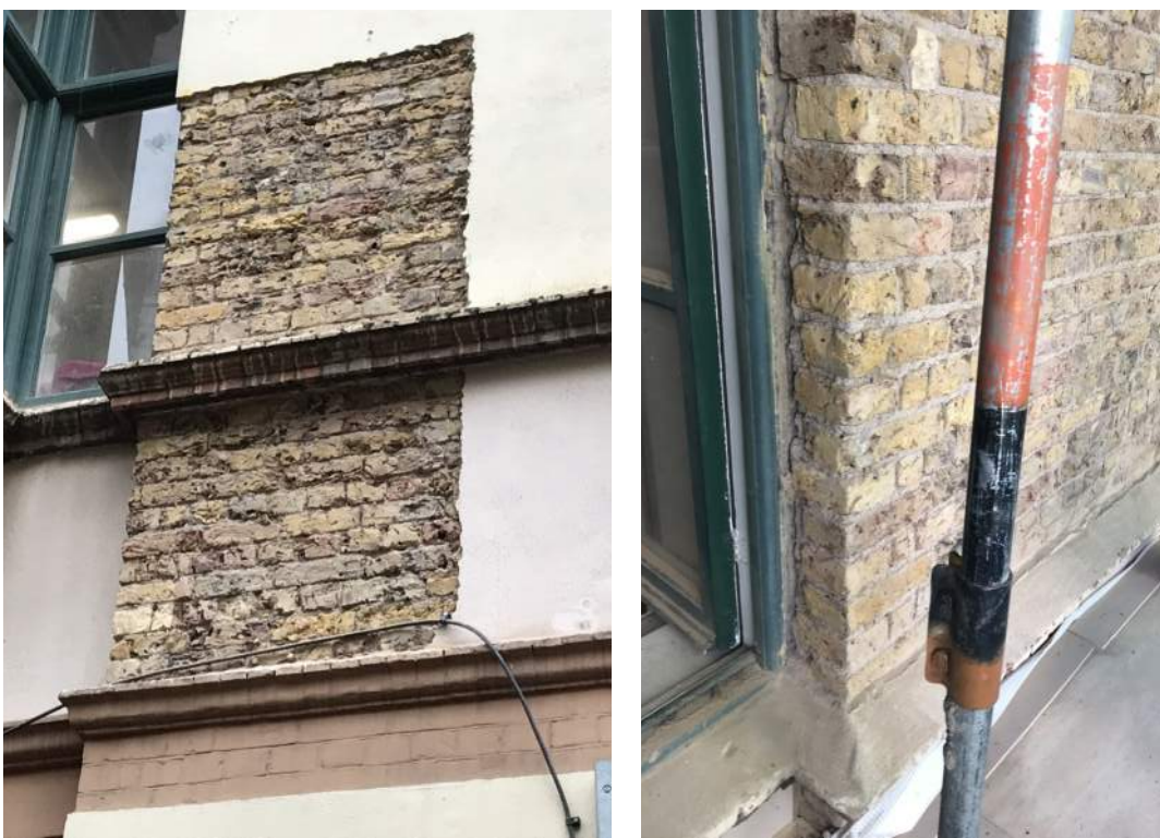
Close-up detail showing render removed - existing stock brick revealed beneath - generally in good condition with light surface damage due to later applied render but brick integrity largely intact. Areas/Bricks with significant damage to be made good in matching brick where the removal has resulted in the loss of the brick surface and would compromise weatherproofing/façade integrity. Mortar joints to be repointed where required
