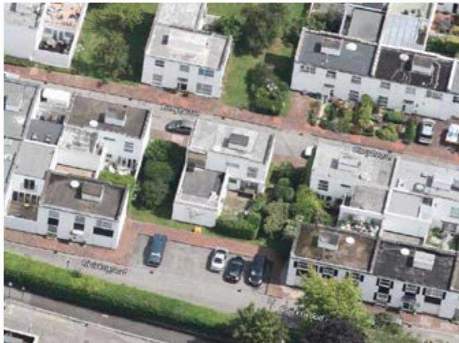
Existing Building - Aerial View West
