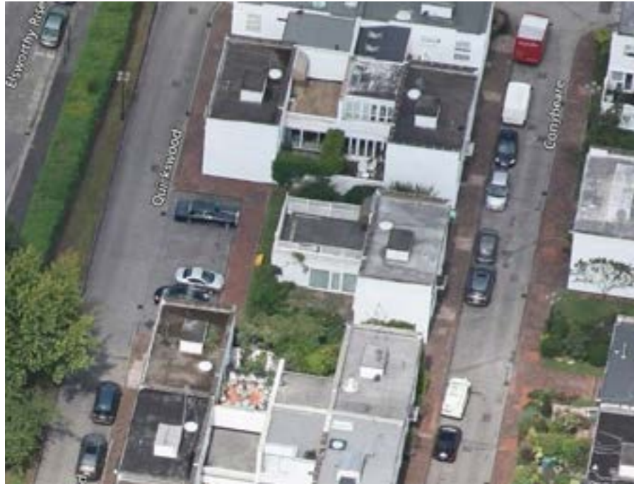
Existing Building - Aerial View North
