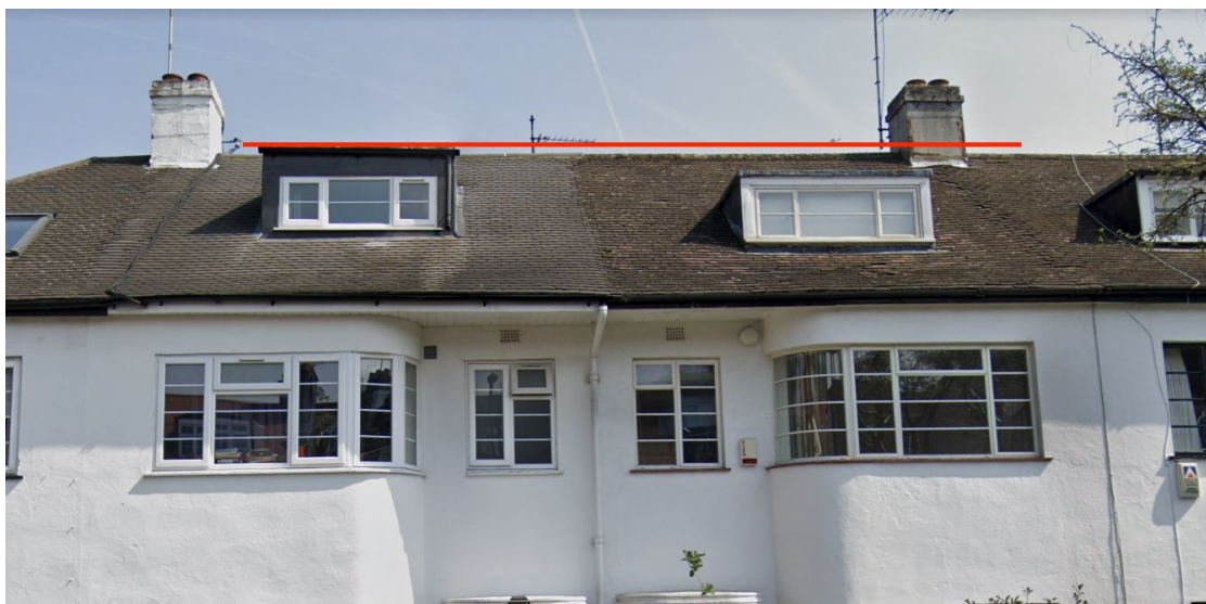
Image of No.78 and 76 Front Elevations
