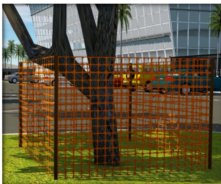
Figure 1: Illustration of Vertical Tree Protection Barrier
