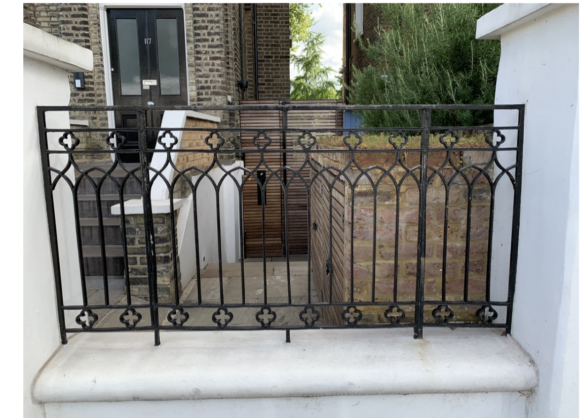
REFERENCE IMAGE: 1100mm H NEW CAST IRON FENCE TO BE INSTALLED ON TOP OF EXISTING RETAINING WALL - DESIGN INTENT
