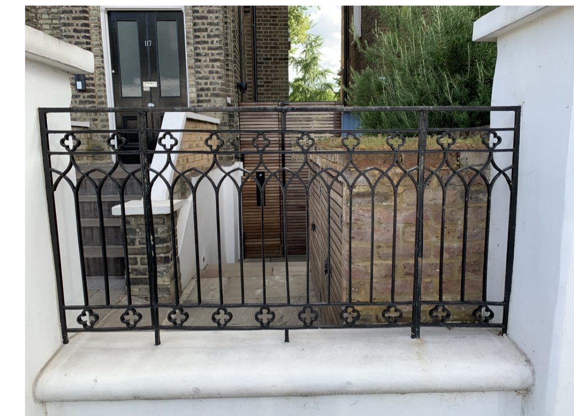
REFERENCE IMAGE: NEW CAST IRON FENCE - DESIGN INTENT PLEASE NOTE: TO BE INSTALLED BOTH AT THE FRONT AND ON THE SIDE BETWEEN PROPERTY no.121 AND no.119
