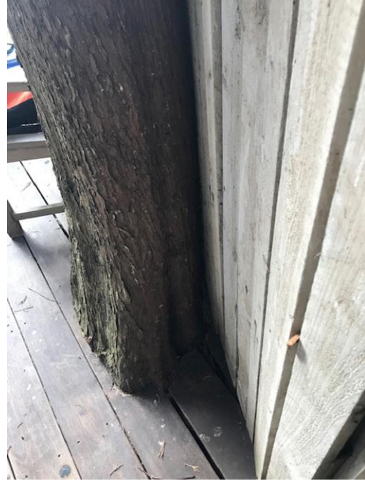
T4- Showing fence proximity
