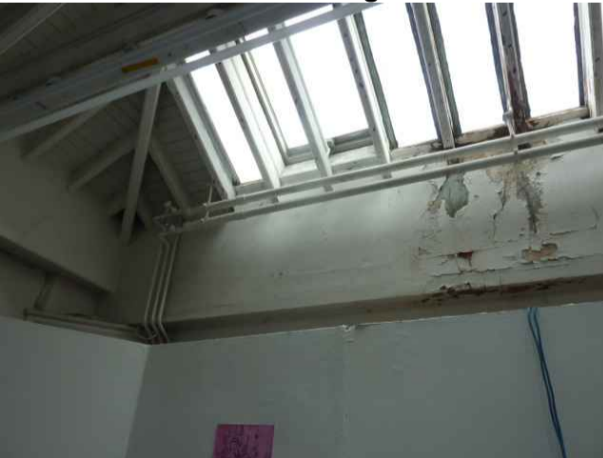
Roof 5 - Internal Glazed Lights
