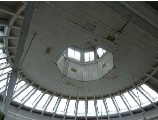
Roof 5 - Internal Dome
