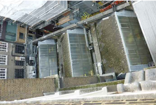
Roofs 9, 11 & 12 – Glazed Lights
