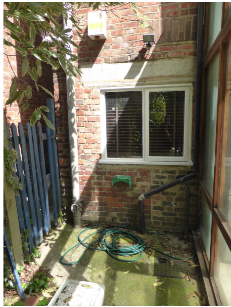
Rear of no.36 including gate to side passage which forms access to land to rear of gardens
