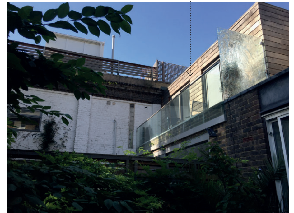
View from the Garden of 10b to the Rear of 9, 10 and 10a Wavel Mews
