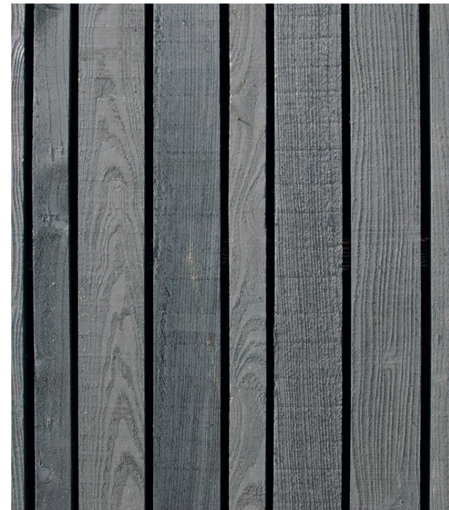
Vertical timber cladding to side extension ①
