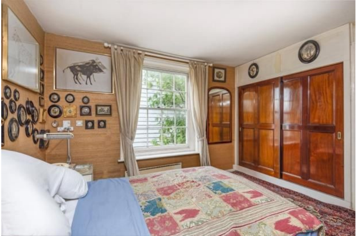
First floor front room: modern Hessian wallpaper to be replaced with skimmed plasterboard lining. Single glazed timber sash windows to be repaired, overhauled and redecorated.
