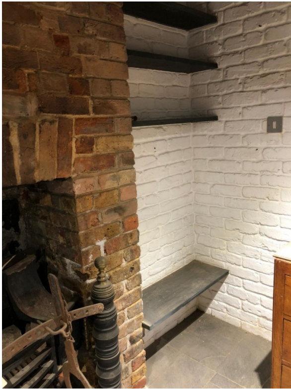
Basement room: previously reception, proposed use as kitchen. Modern timber ceiling to be removed. Existing fireplace: to be adjusted to suit new kitchen installation (raised plinth to be removed, arch head to be raised, slate shelves to be removed)
