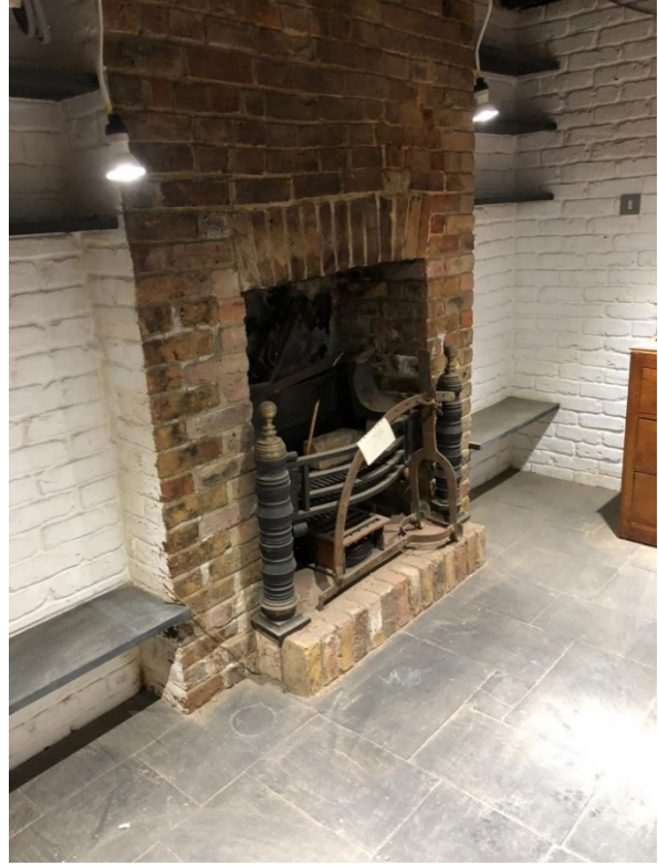
Basement room: previously reception, proposed use as kitchen. Modern timber ceiling to be removed. Existing fireplace: to be adjusted to suit new kitchen installation (raised plinth to be removed, arch head to be raised, slate shelves to be removed)
