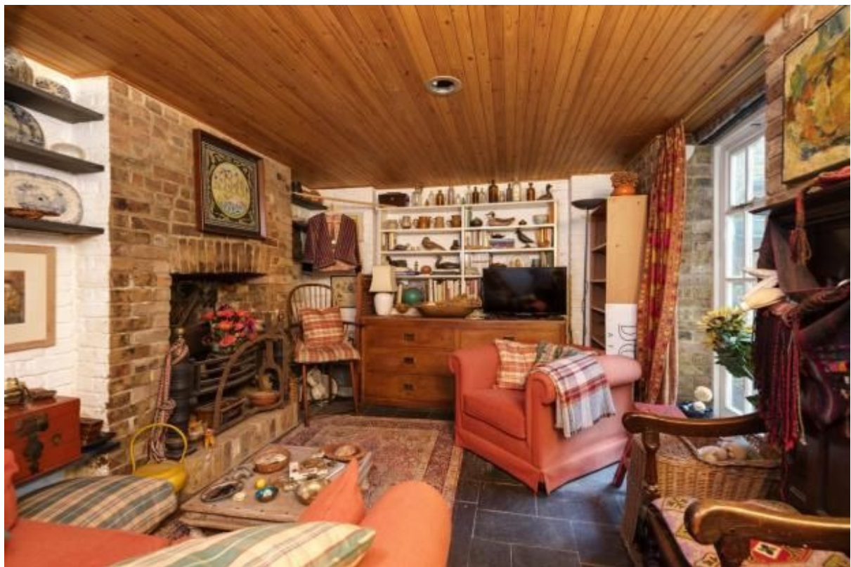
Basement room: previously reception, proposed use as kitchen. Modern timber ceiling to be removed. Existing fireplace: to be adjusted to suit new kitchen installation (raised plinth to be removed, arch head to be raised, slate shelves to be removed)
