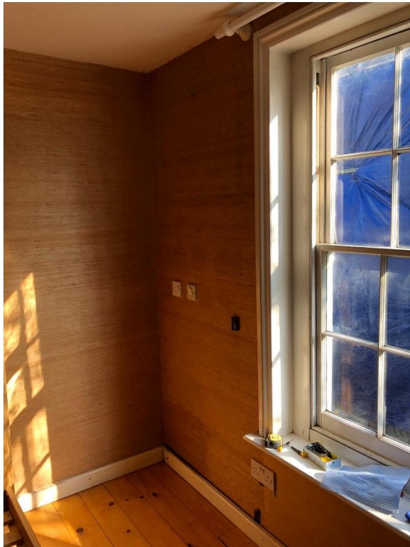
First floor front room: modern Hessian wallpaper to be replaced with skimmed plasterboard lining. Single glazed timber sash windows to be repaired, overhauled and redecorated.
