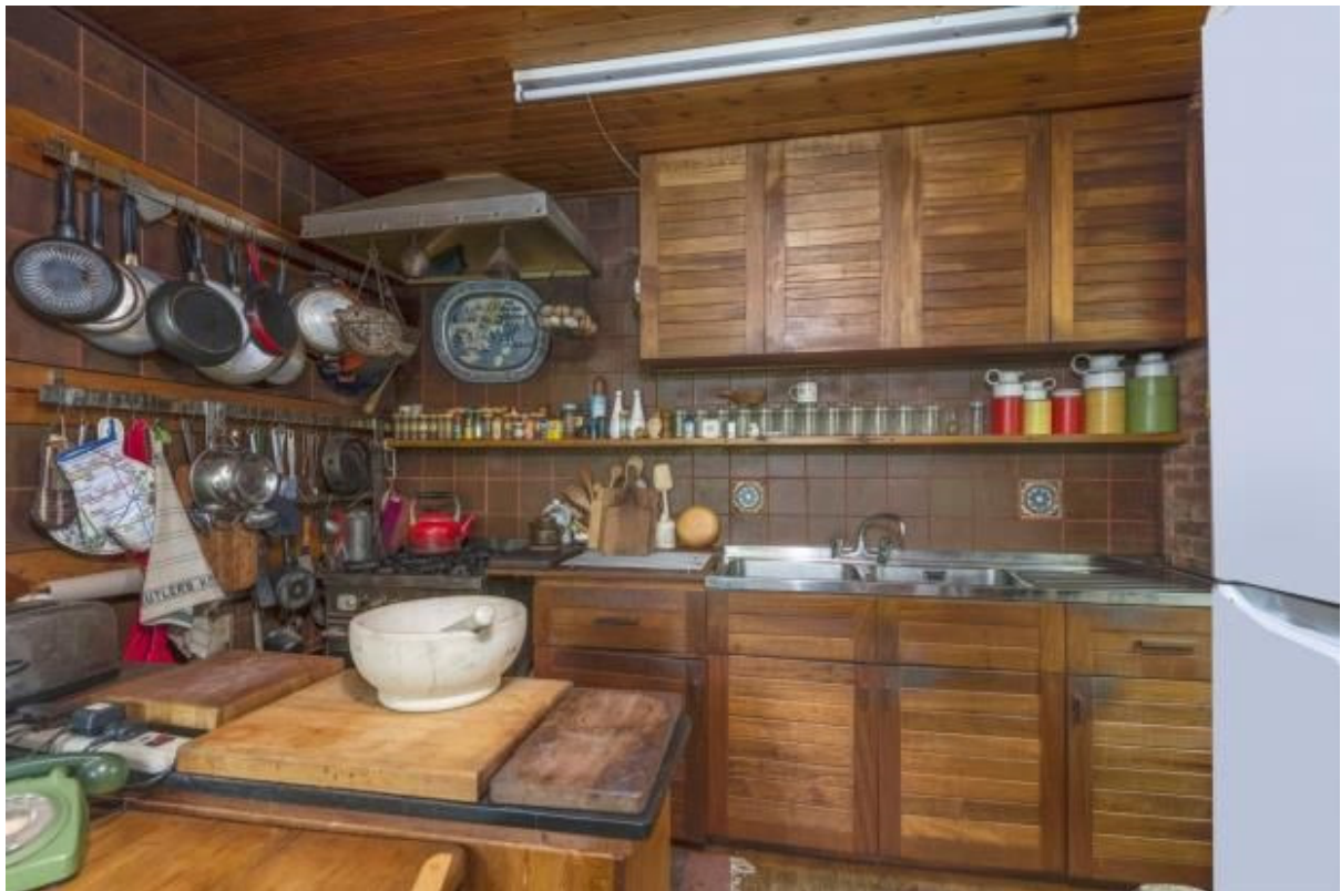
Modern first floor rear extension: existing kitchen fittings, timber board wall and ceiling lining to be removed.
