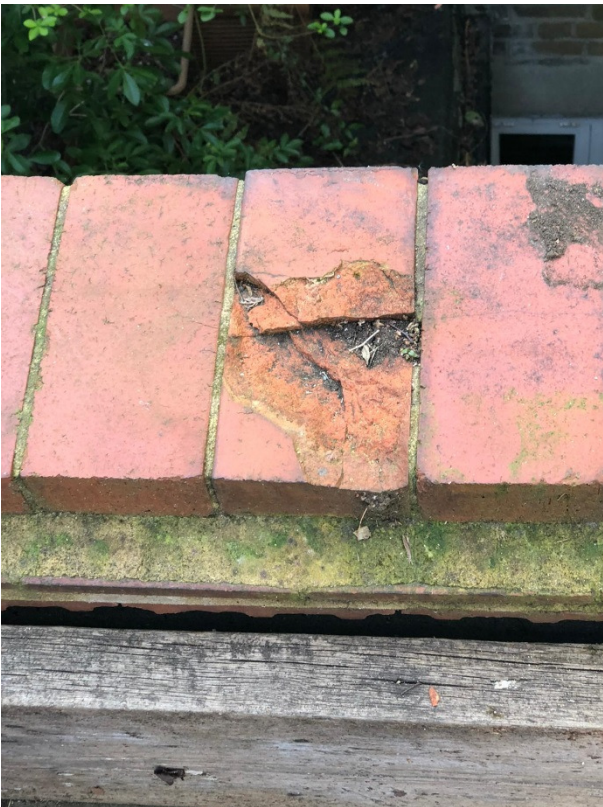
Above: rear roof terrace Below: damage to parapet wall to be repaired Below right: second floor room rear door to roof terrace
