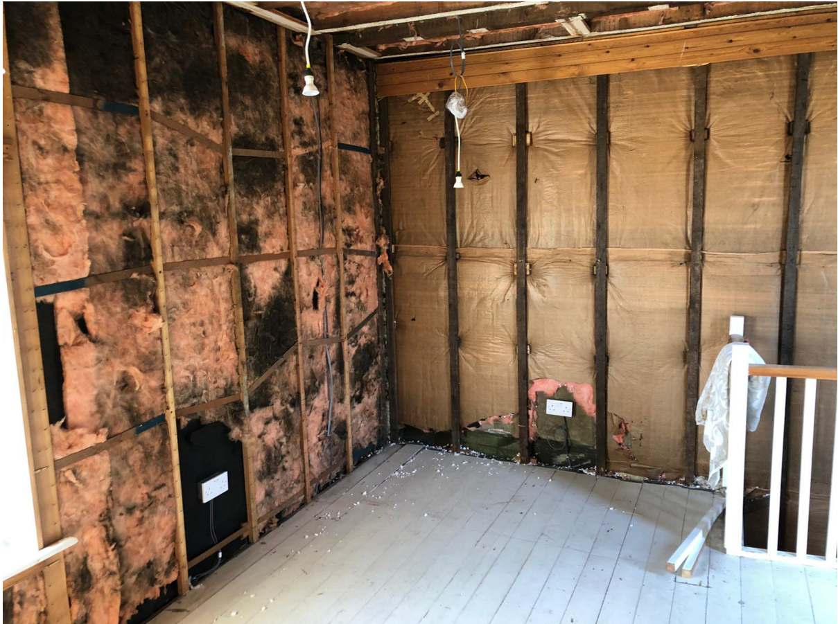
Second floor room: before removal of modern timber board cladding to walls and ceiling (photo above) and after removal of cladding carried out for re-wiring and due to damp.
