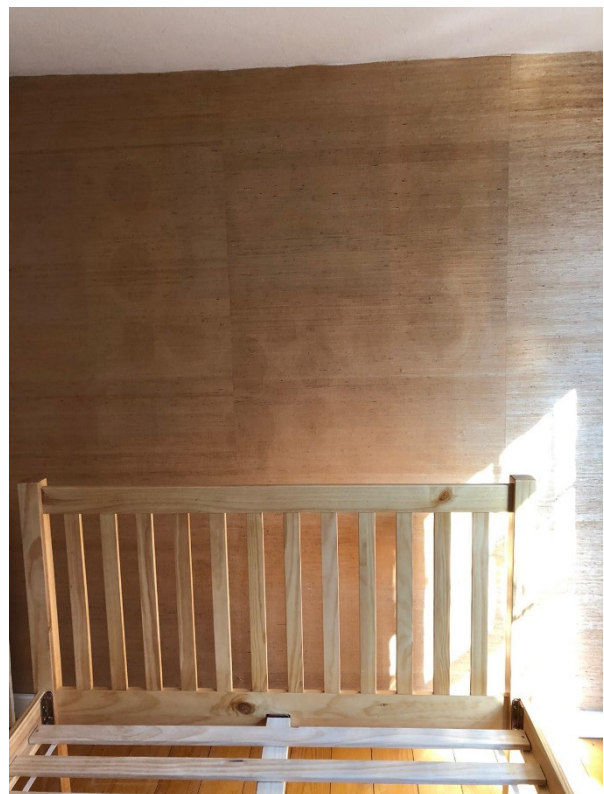
First floor front room: modern Hessian wallpaper to be replaced with skimmed plasterboard lining. Single glazed timber sash windows to be repaired, overhauled and redecorated.
