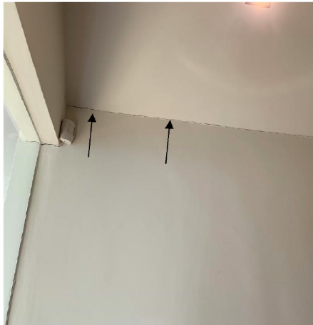
Hall - shrinkage crack
