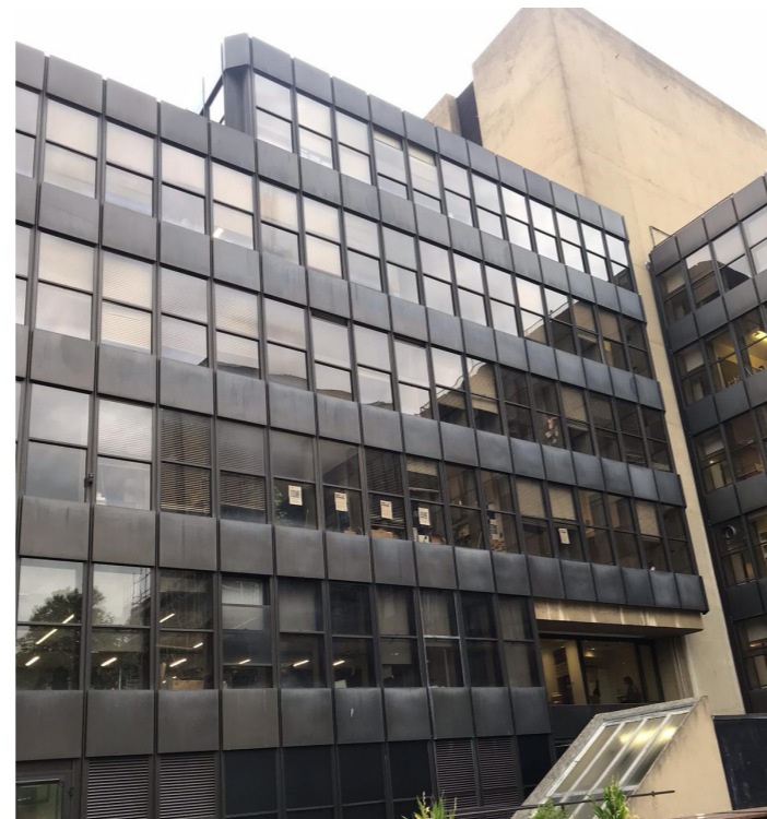
Photograph of existing elevation
