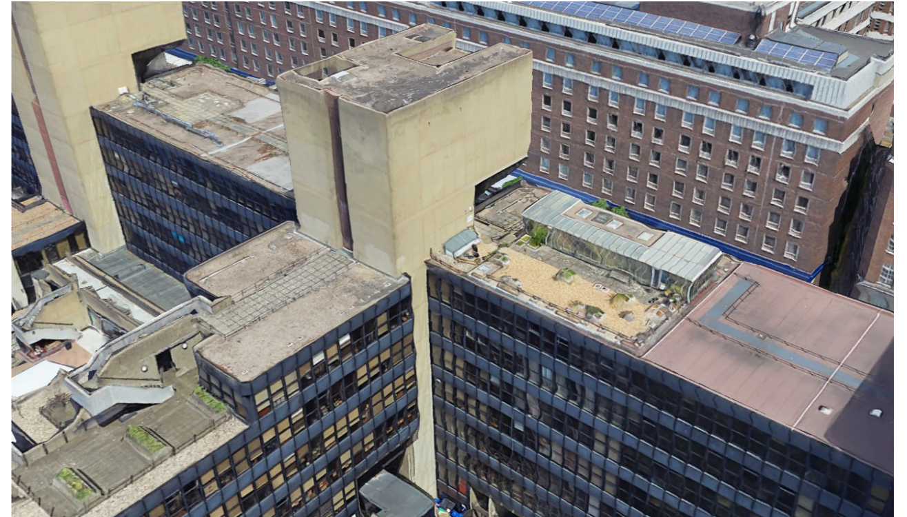
Existing Level 10 roof
