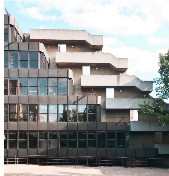
View of the Northern side of the Wing - Level 5
