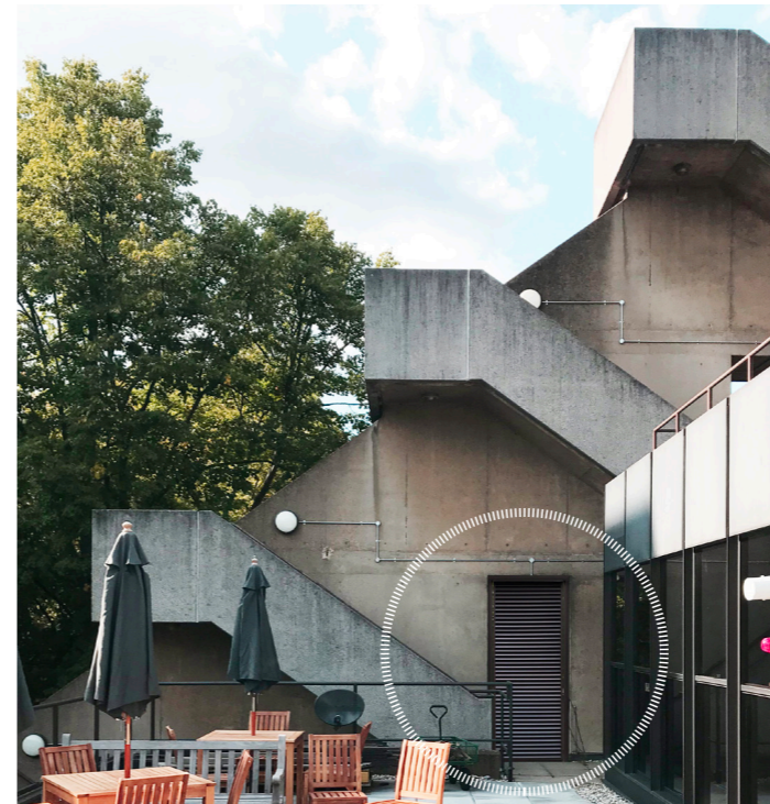
Louvred gate to existing opening - View from level 5 terrace
