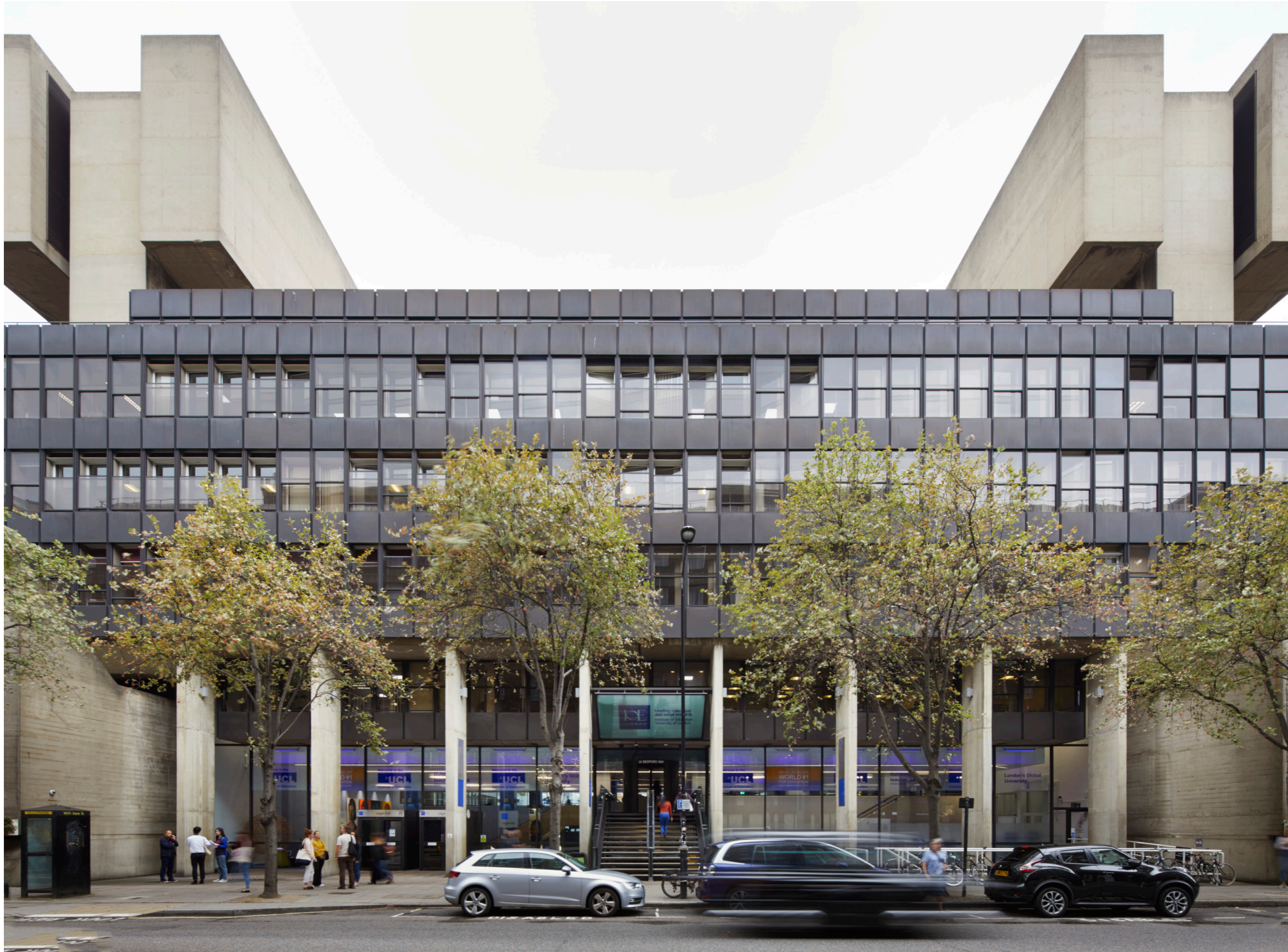
Photograph from Bedford Way
