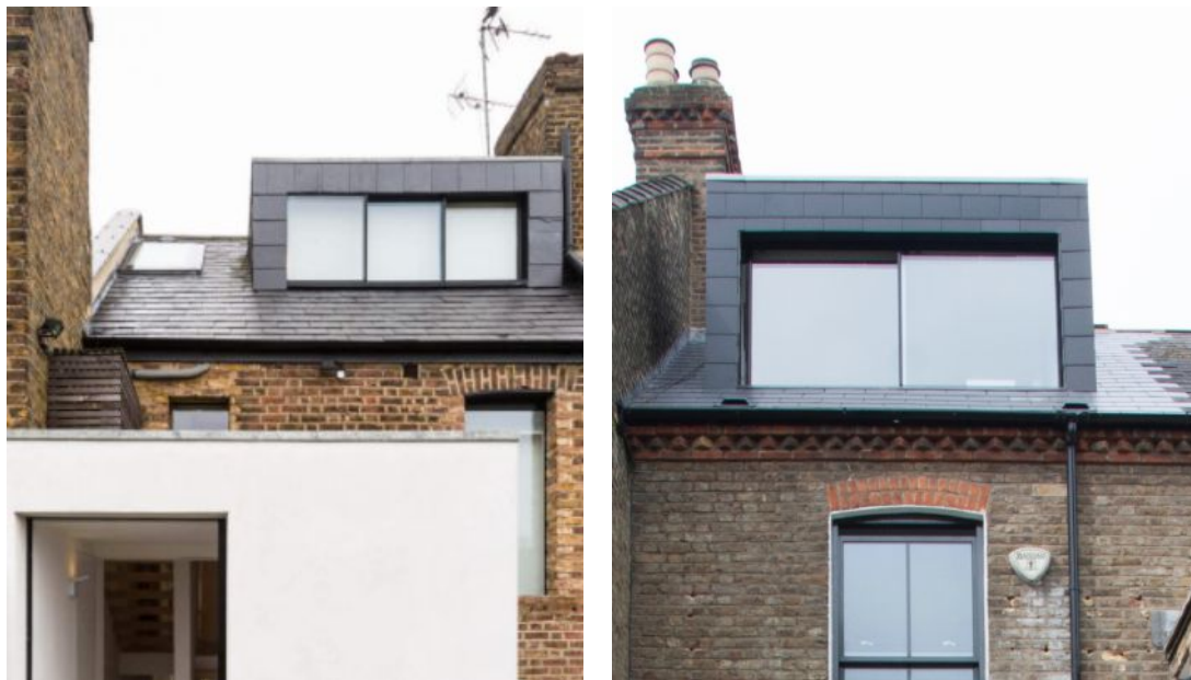
Fig. 01 examples of dormer extensions designed by William Tozer Associates, in conservation areas, using contextual materials and minimal glass framing.
