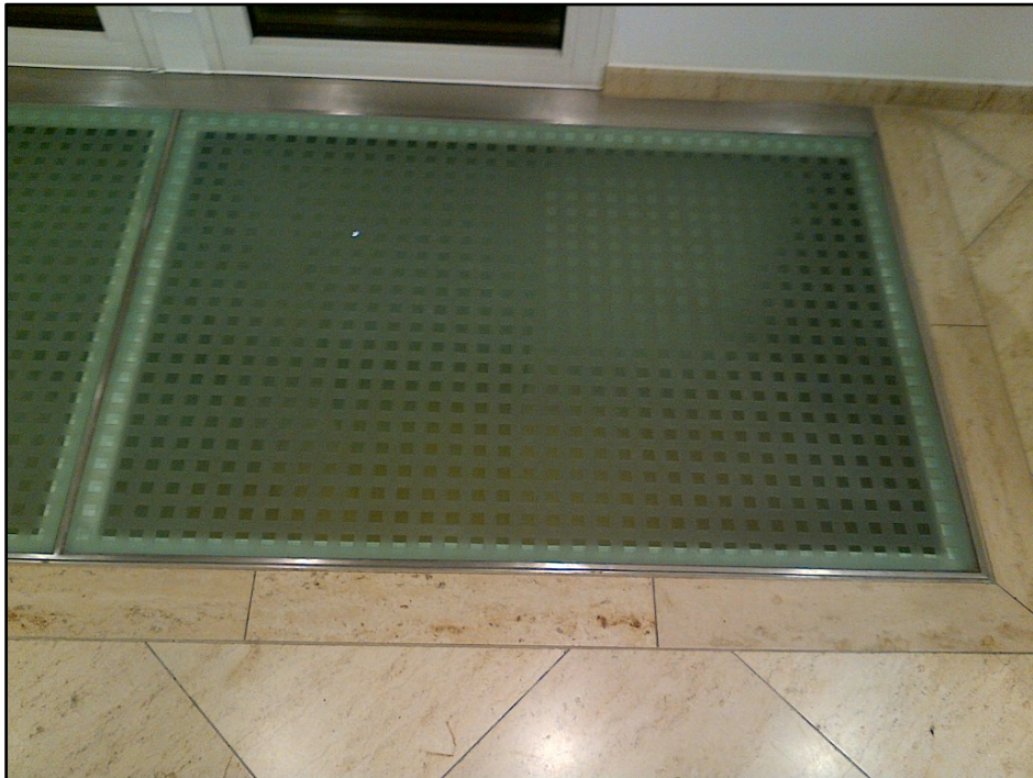
Photo 7: Example of Lightwell Screen Glazing 1.
