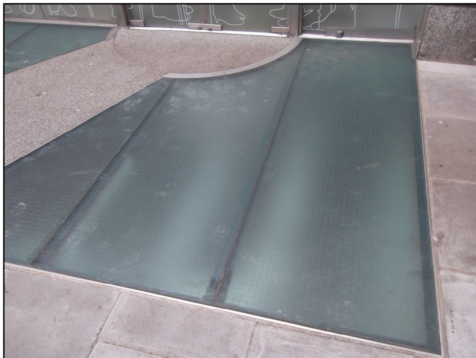
Photo 8: Example of Lightwell Screen Glazing 2.
