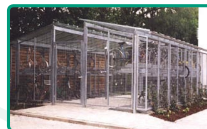
Berlin shelter - lockable compound
