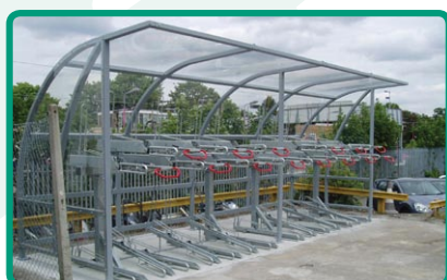
Solent extended shelter (Upminster station)
