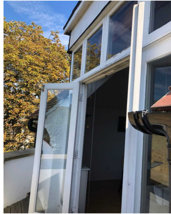
Existing timber French doors showing projecting element of the roof into balcony zone
