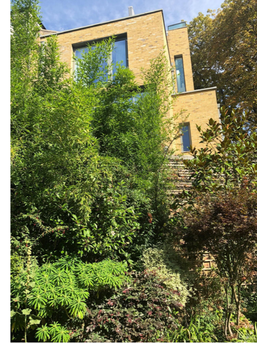
Contemporary neighbouring property to north of the boundary with large aluminium framed windows
