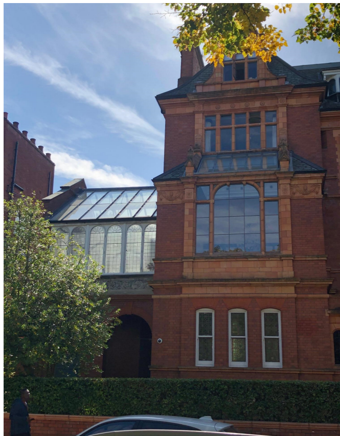
Eaton Avenue - example of timber framed sash windows at low level, with light framed highly glazed areas above and roof level glazing.
