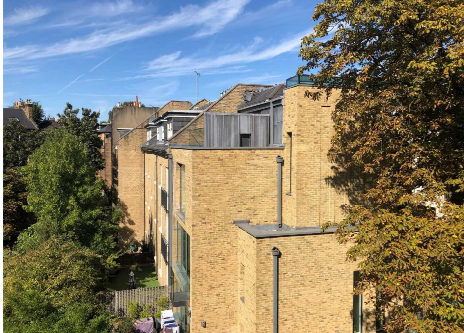
Contemporary neighbouring property on Lancaster Grove with structural glazing and zinc cladding at high level
