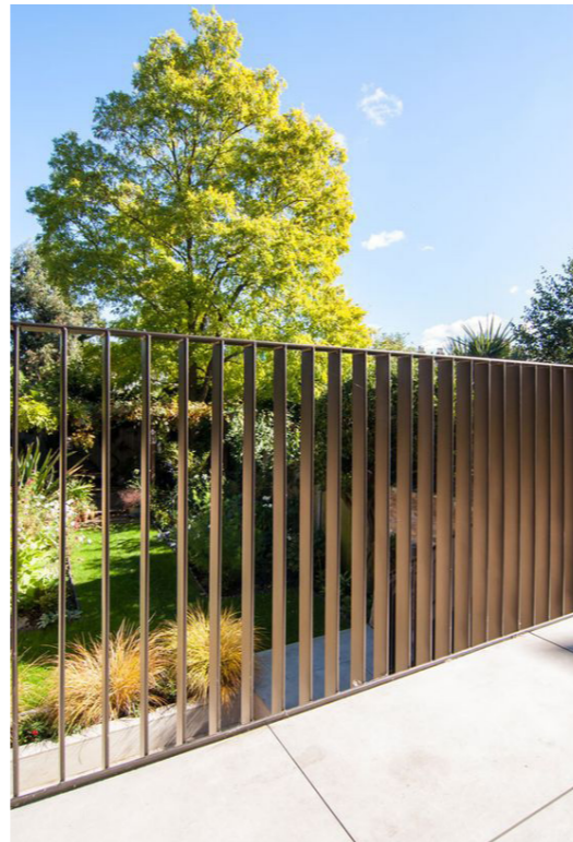
Simple wrought iron balustrade
