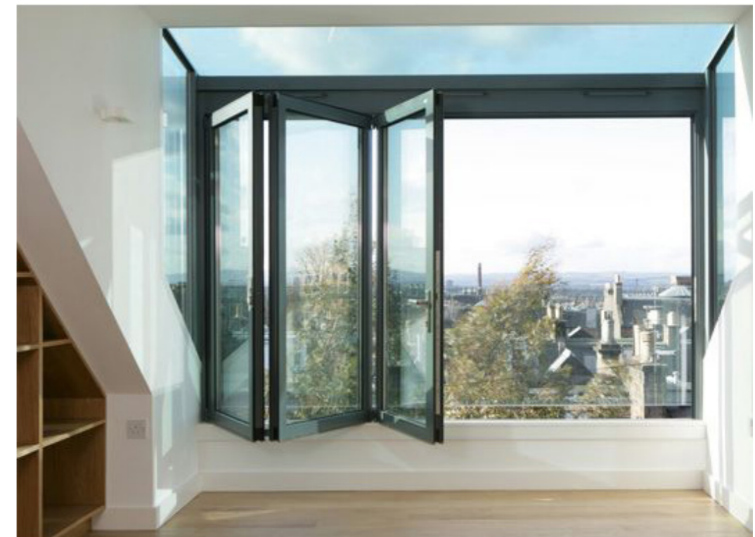
Slim line inward opening aluminium bi-fold doors with fixed side lights and roof glazing
