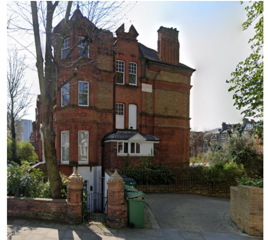
North elevation of 2 Strathray Gardens from Lancaster Grove
