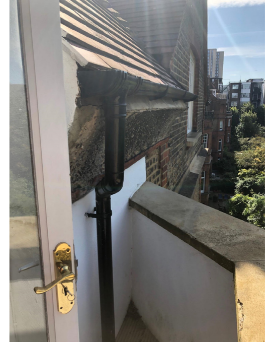
Existing drainage outlet on to roof
