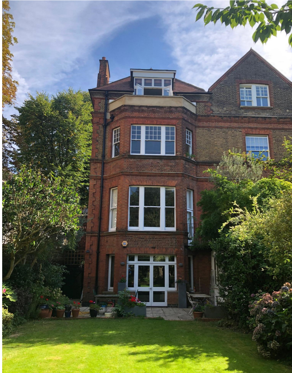
Existing west elevation - Dormer construction with French doors to the third floor apartment.
