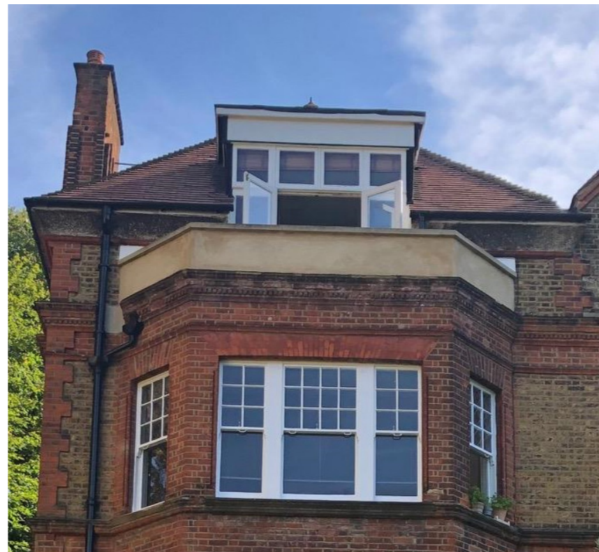
Existing timber French doors showing projecting element of the roof into balcony zone
