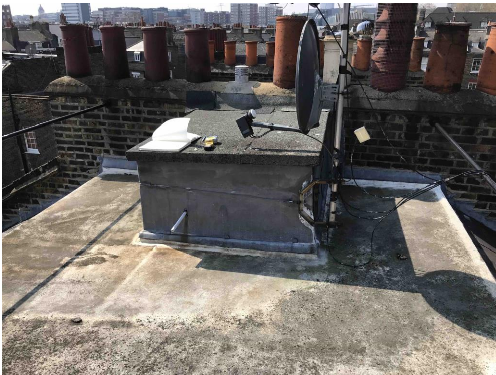
3 Wren Street main roof flat portion looking west
