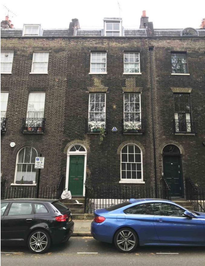
3 Wren Street front façade
