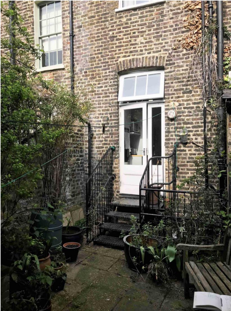
3 Wren Street rear ground level access via kitchen
