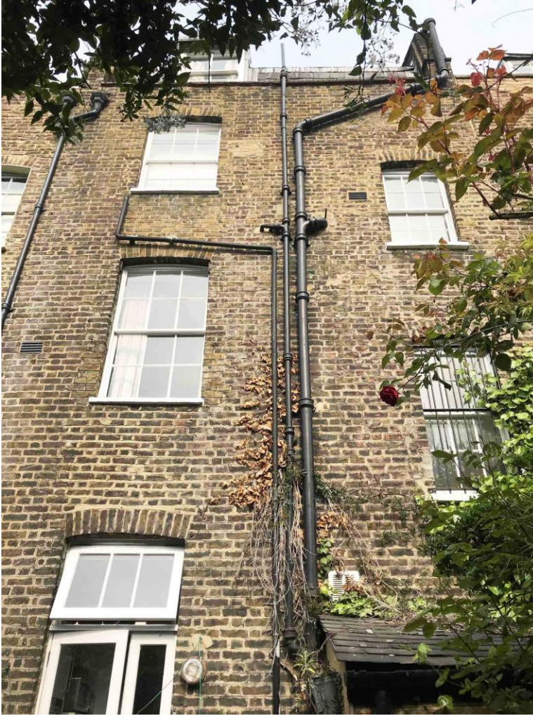
3 Wren Street rear façade
