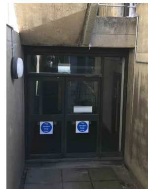
6 Rear Wing Existing Door Level 6,7 &8 PHOTO NS
