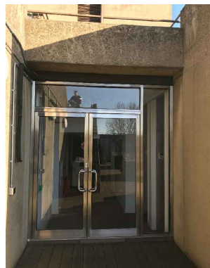
5 Rear Wing Existing Door Level 9 PHOTO NS
