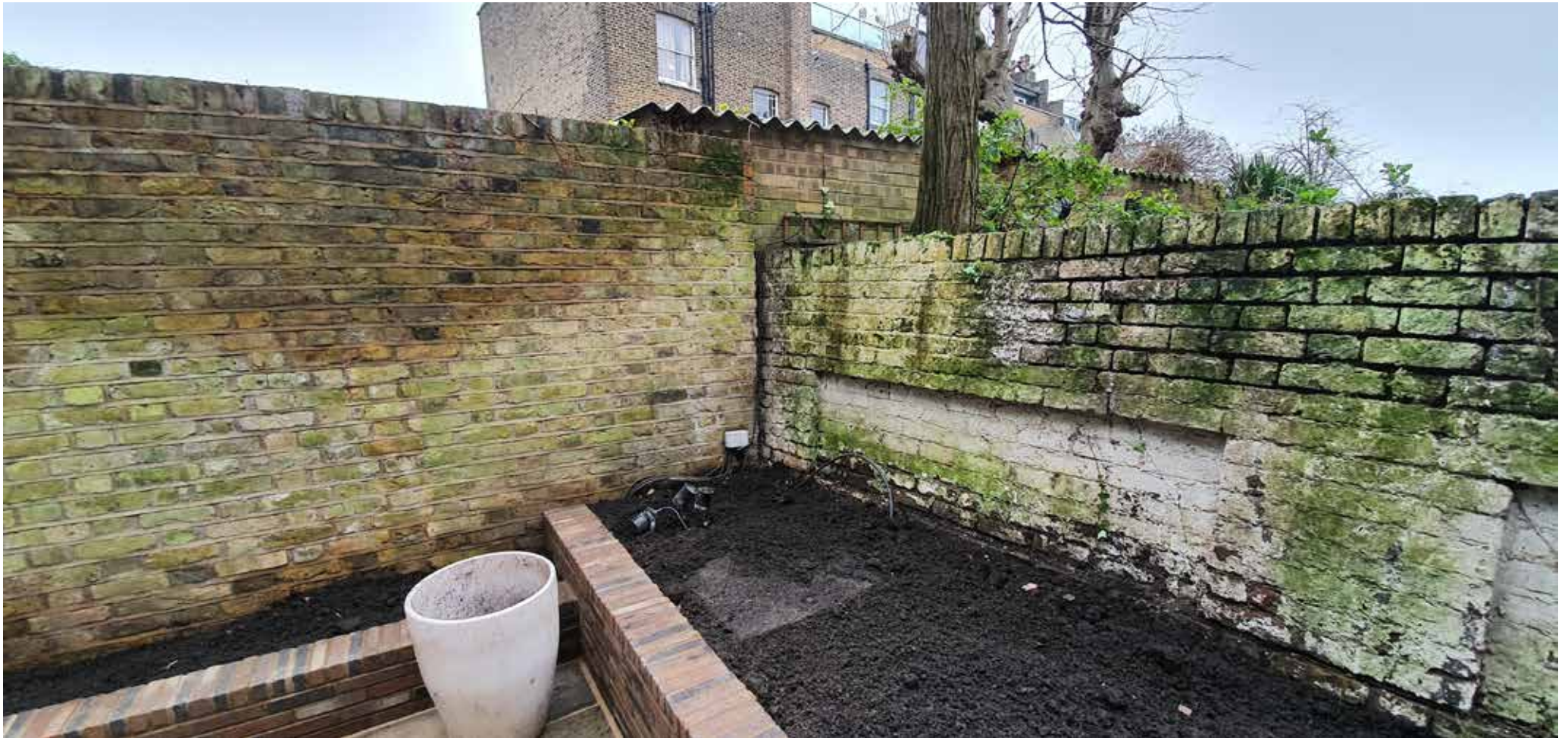
Existing Rear Garden : The proposed Eco-Playhouse will be site in the bottom right side (South East) corner of the garden
