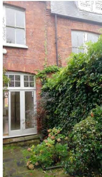
VIEW TOWARD BOUNDARY WITH NO. 24: NOTE HEIGHT AND DENSITY OF VEGETATION ON GARDEN BOUNDARY FENCE
