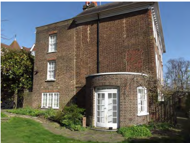
11 Western elevation of Vine House includes a larger, but single bow front and evidence of bricked-up windows on the first and second floors, view east
