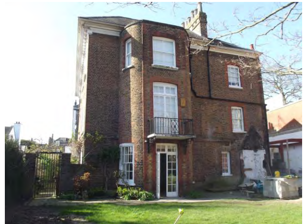
10 Eastern elevation of Vine House dominated by its double bow front and evidence of the former glass house extension, view west
