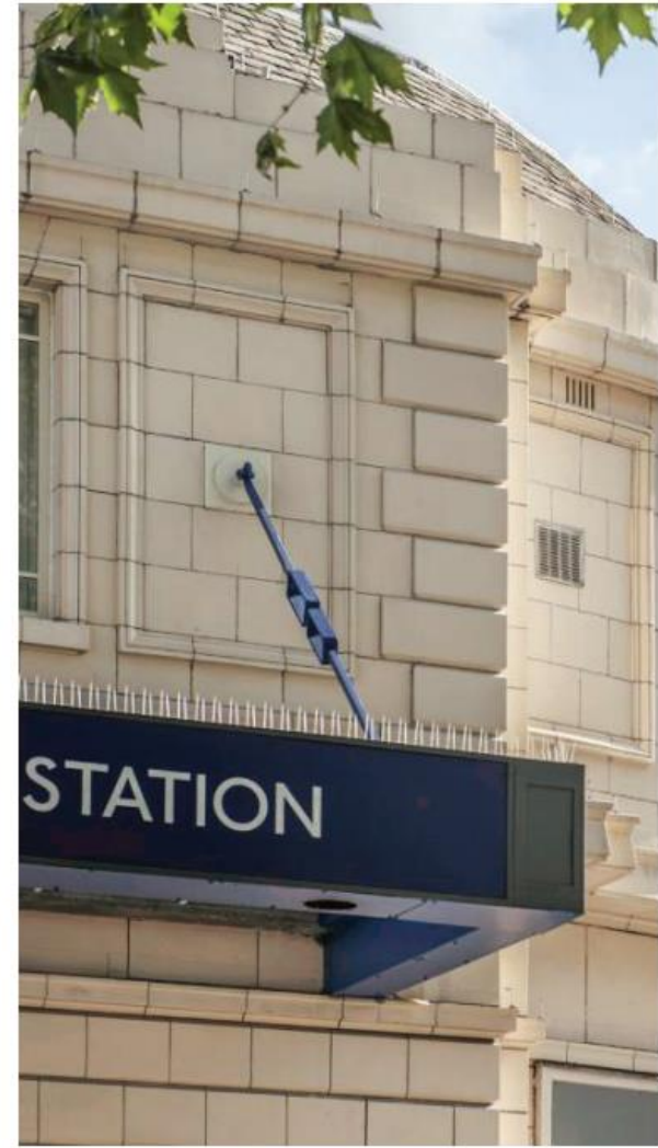
Figure 41 Use of Faience, Great Portland Street LU Station
