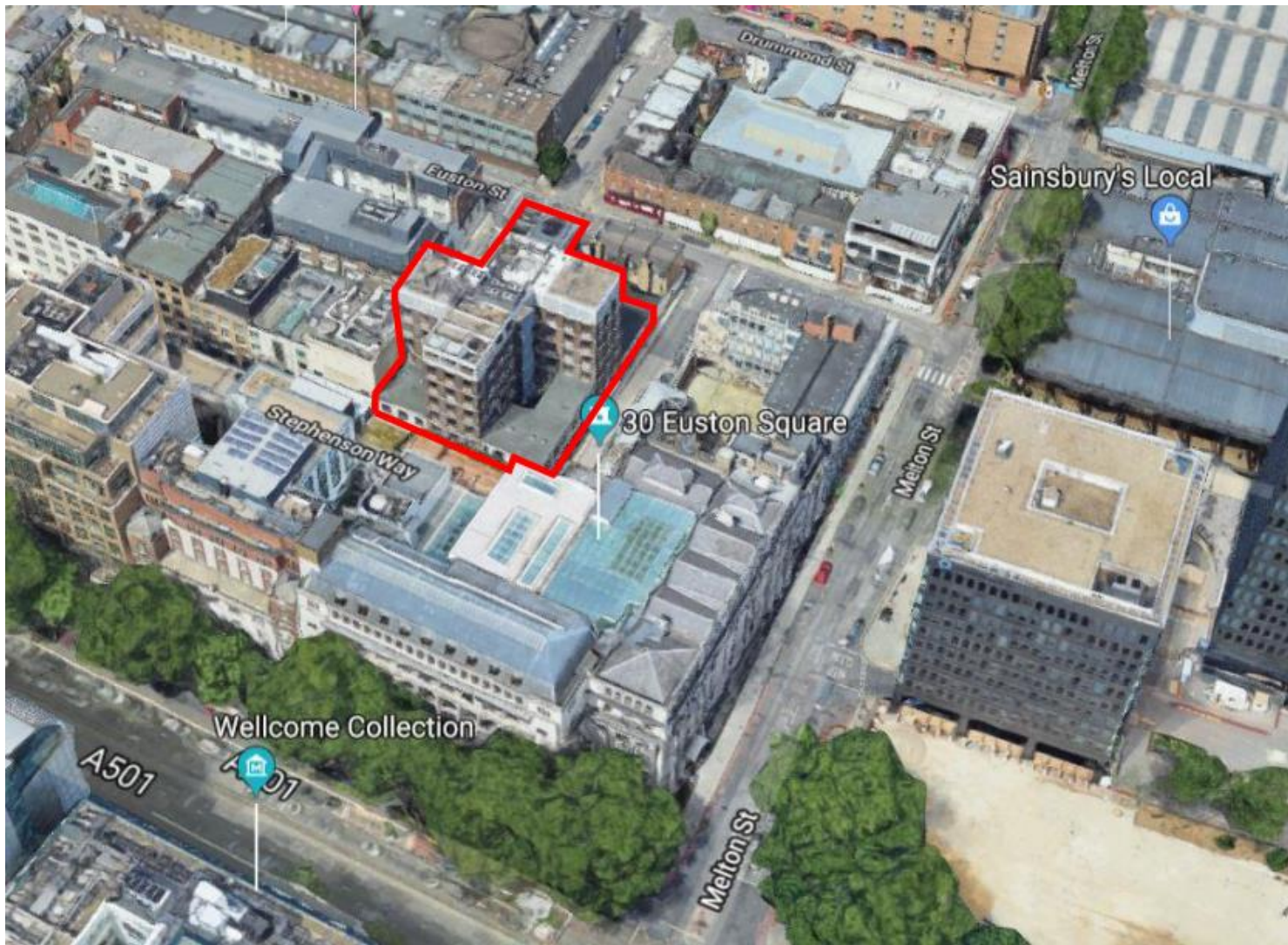
Aerial view of existing building to be demolished (Wolfson House)
