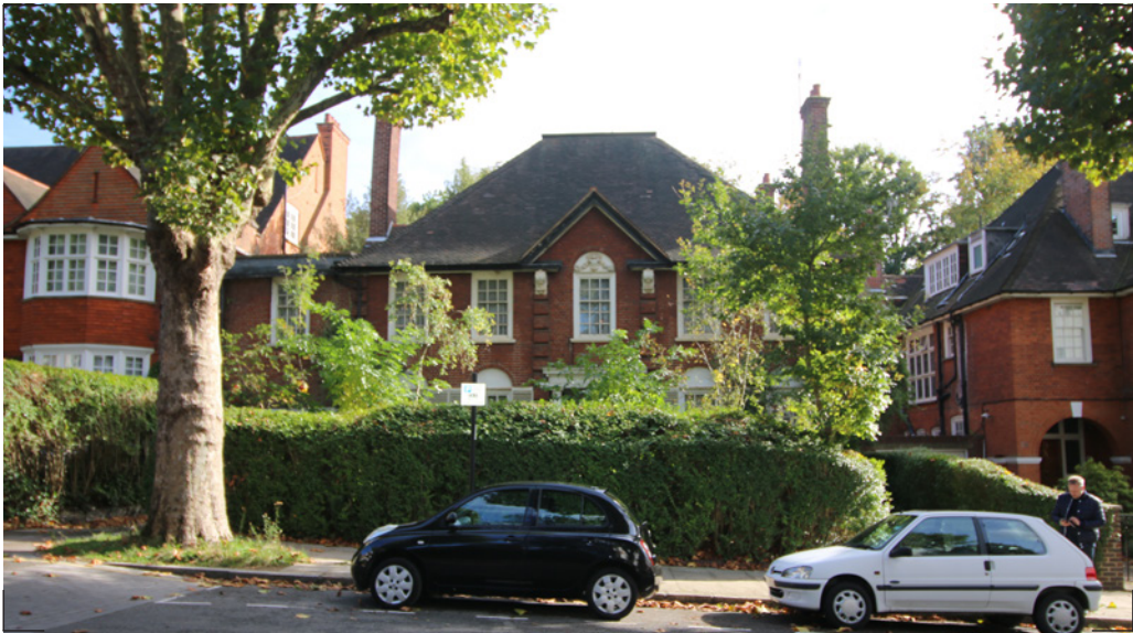
EXISTING CHIMNEY PRE STORM.
