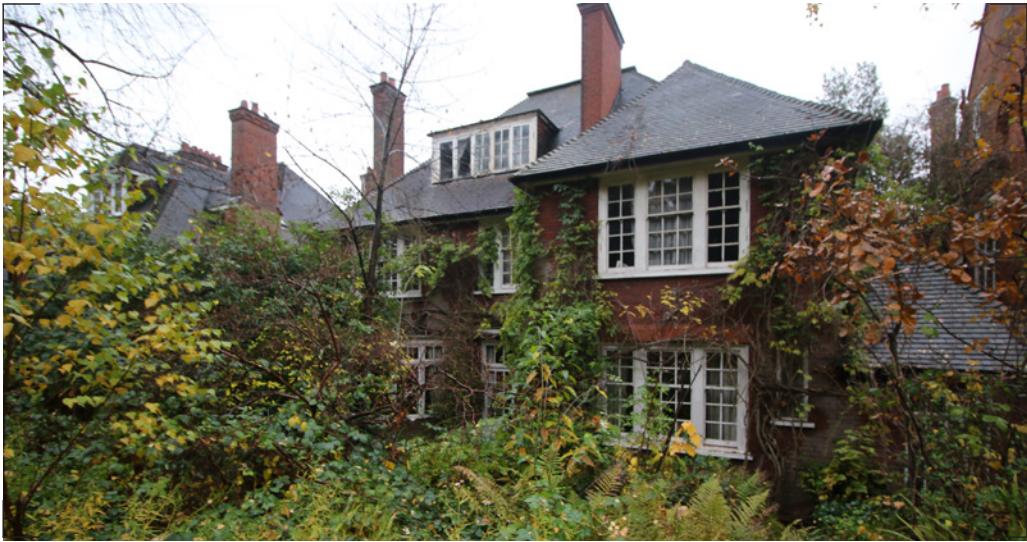
EXISTING CHIMNEY PRE STORM.
