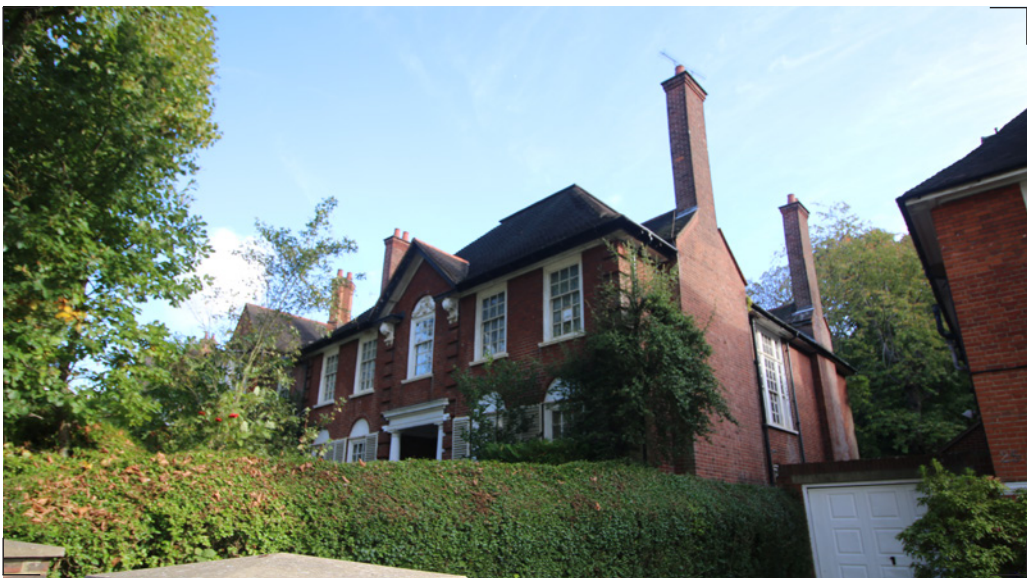
EXISTING CHIMNEY PRE STORM.
