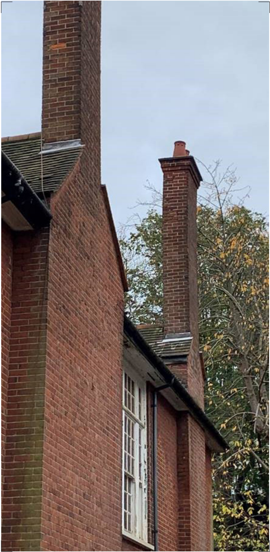
EXISTING CHIMNEY POST STORM.
