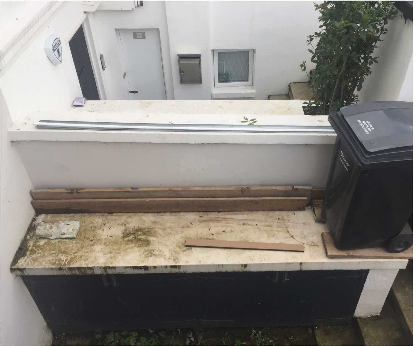
PHOTO 4 - Existing bin shed
