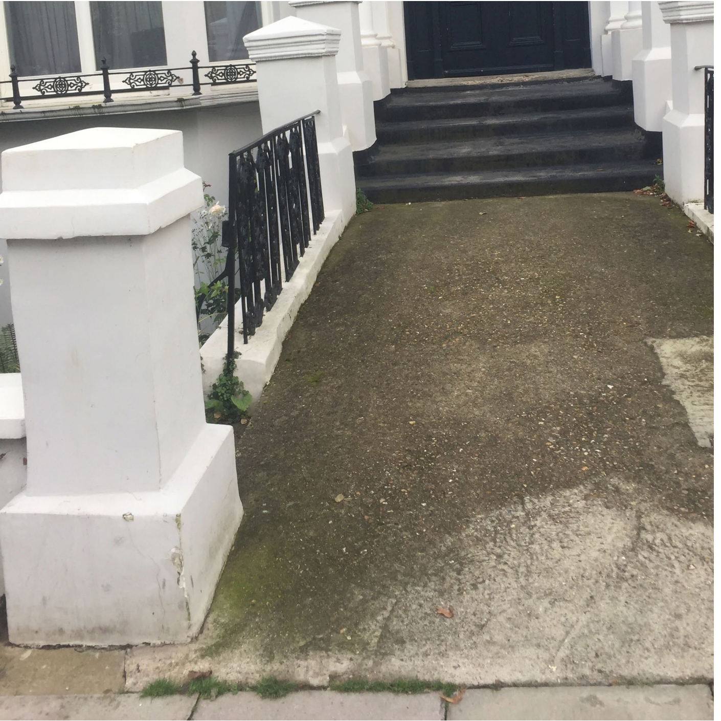
PHOTO 5 - Existing entrance paving
