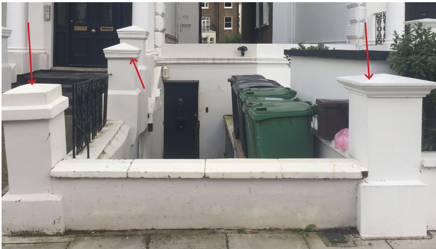
PHOTO 2 - Piers with different shape of caps
