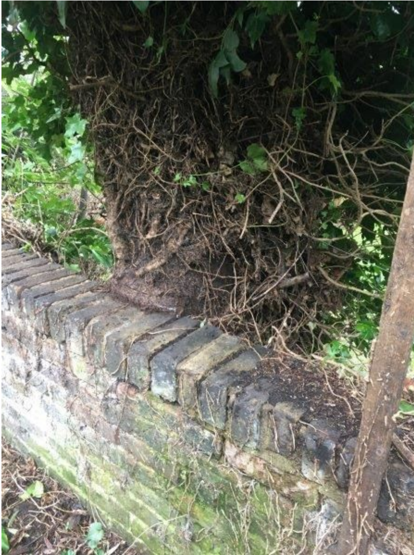
Photo 5: T3 Large trunk pushing against boundary wall
