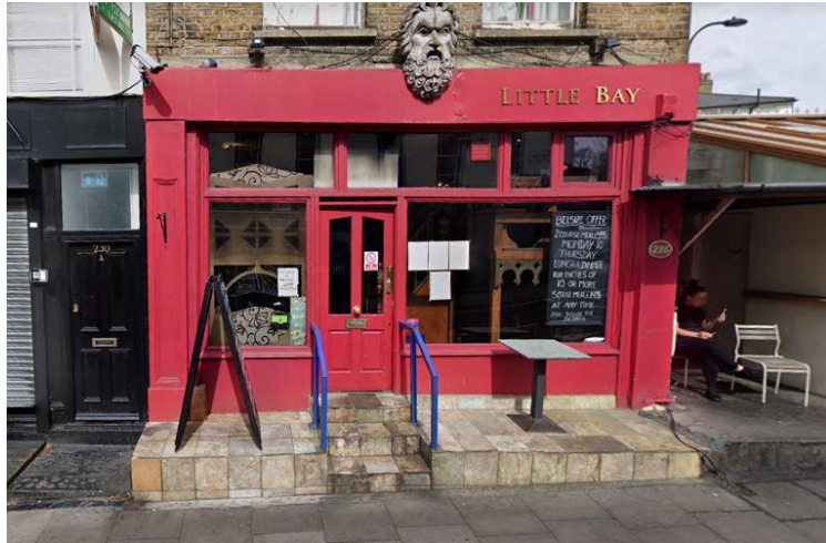
Figure 3. Existing Front Elevation Door
