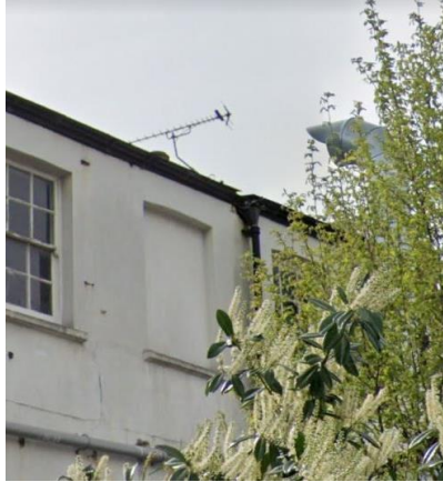
Figure 5. Existing and Approved 2nd Floor Blocked Rear Window
