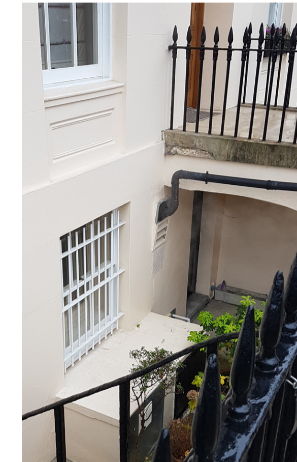
LOUVRES IN NO. 33 CHESTER TERRACE FRONT LIGHT WELL
