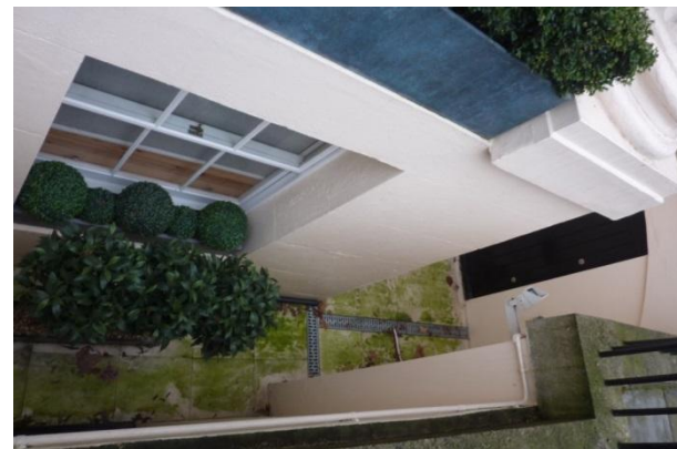
Figure 19: View of No. 36 front light well over railings
