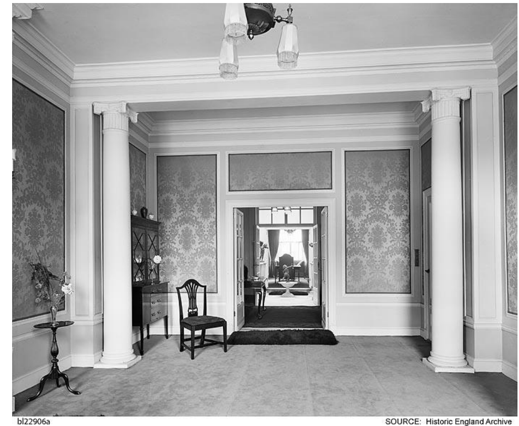
Figure 24: Morning room, Ground Floor, 14 Chester Terrace, 1914, following restoration by R Frank Atkinson. Historic England Archives. The extended form of the front ground floor rooms of Chester Terrace that was in place prior to the introduction of lift shafts is clearly seen. Columns are used to separate the spaces. A double-door opening connects the front and rear rooms. The axis is reinforced through openings to the light well and rear volume beyond.
