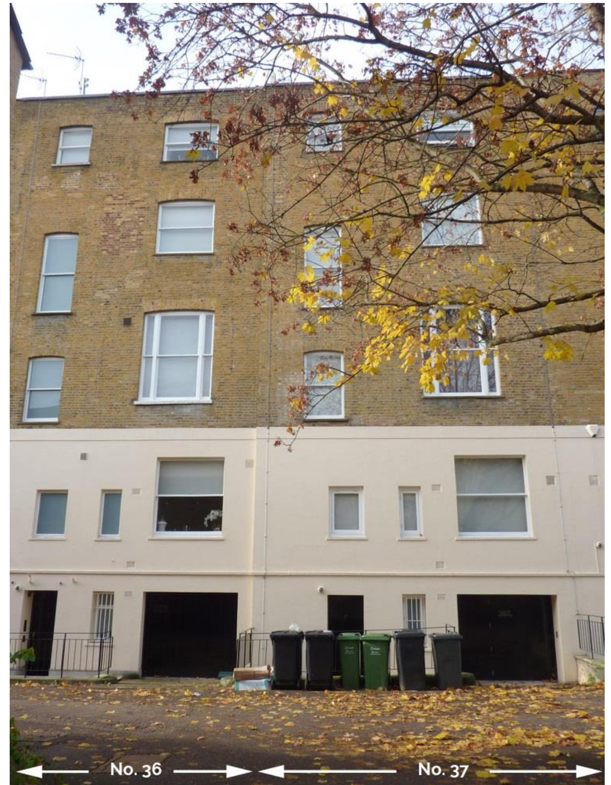
Figure 5: Rear elevations of Nos. 36 & 37 Chester Terrace
