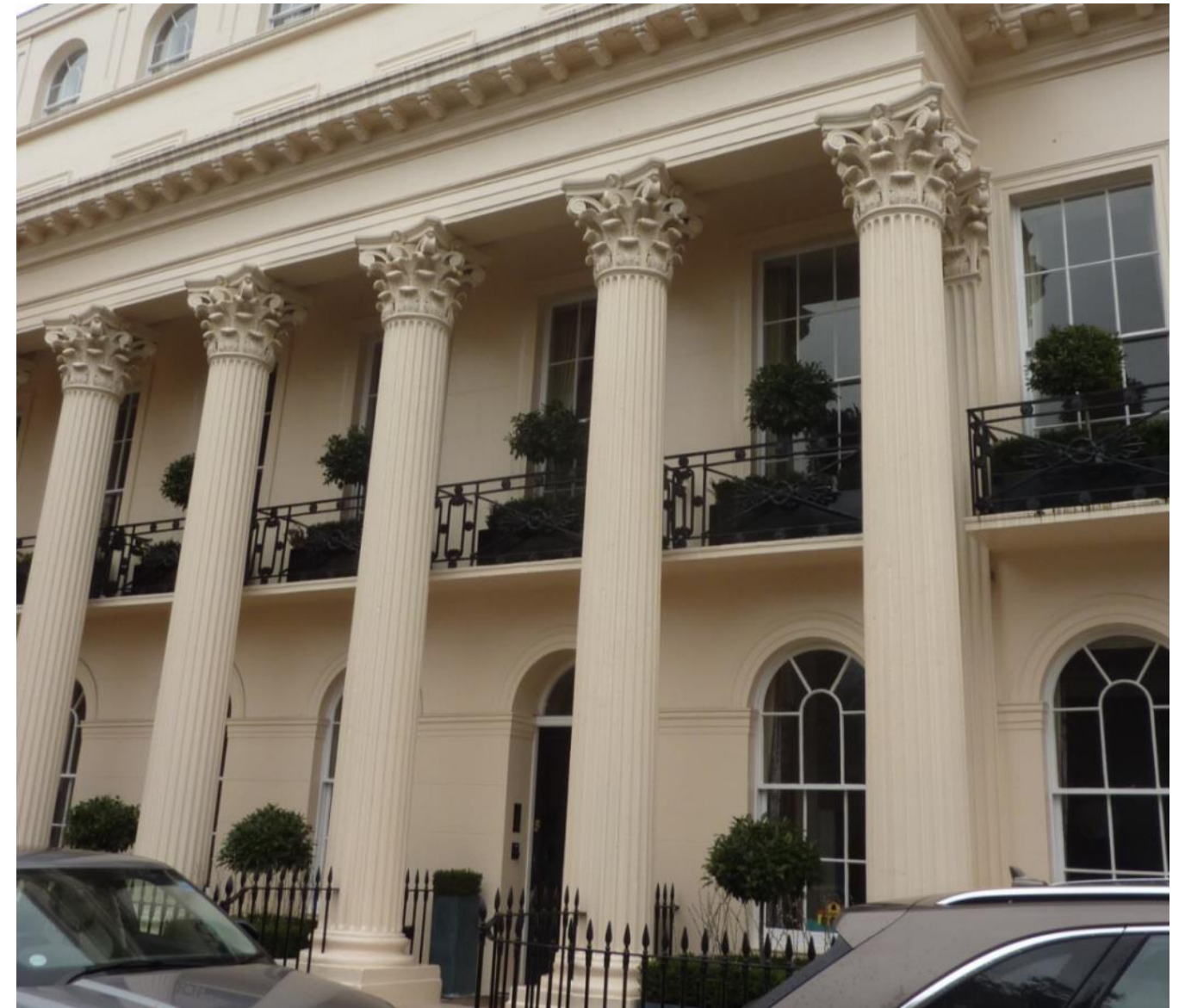
Figure 26: Visibility of proposed opening is obscured by colonnade and deep window reveal
