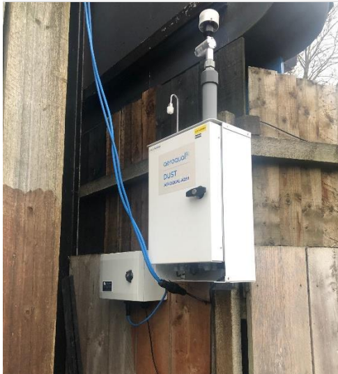
Dust, Noise and NO2 monitor
