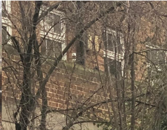
View from St Andrews Garden
