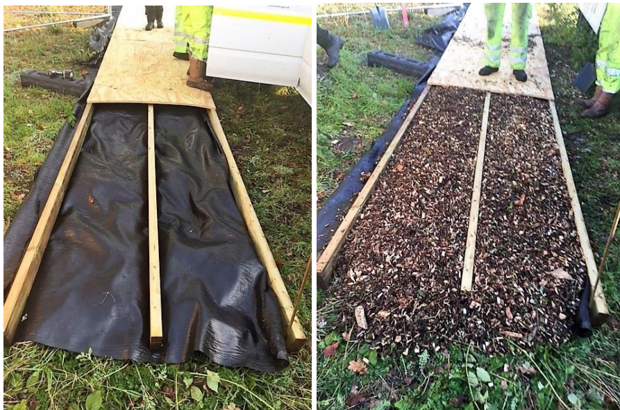
Figure 6. Plywood sheeting used as ground protection.
