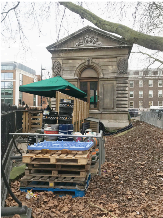
Current obstructed view of north elevation when approaching from Euston
