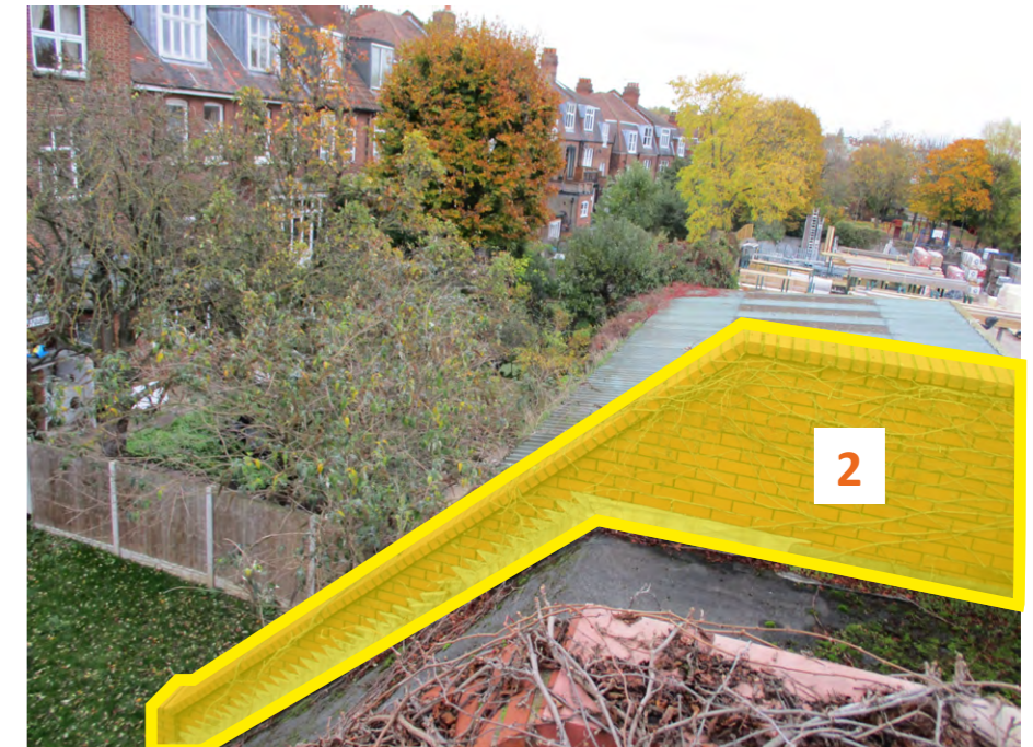
2. Retain brick parapet wall between two chamfered roofs in Phase 1 & 2. To be demolished in Phase 3.
