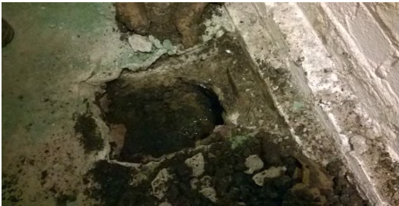
View into TP1 - looking southeast
