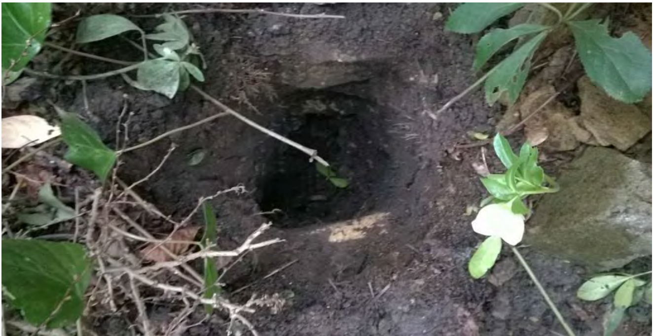
View into TP3 - looking north
