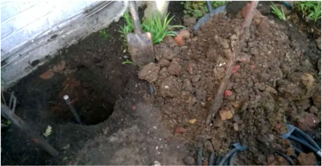
View of TP6 - looking northwest
