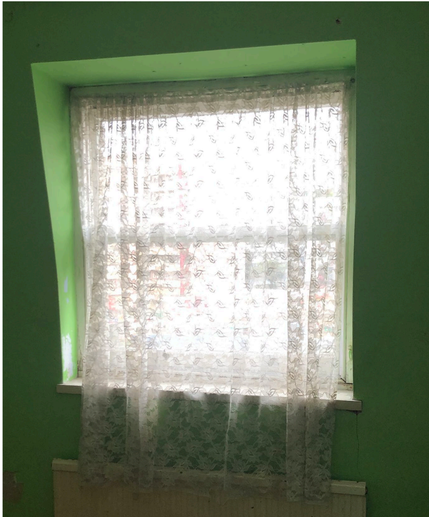
Figure 9: Internal view of window at third floor level – bedroom
