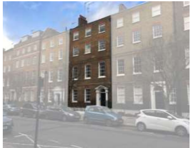
Fig.02 Looking north along John Street
