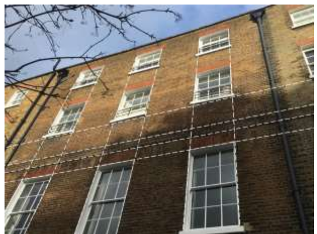
Fig.04 Grid mark-up showing distortion
