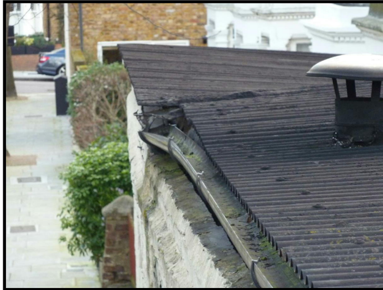
PHOTOGRAPH 3 – Defective guttering.
