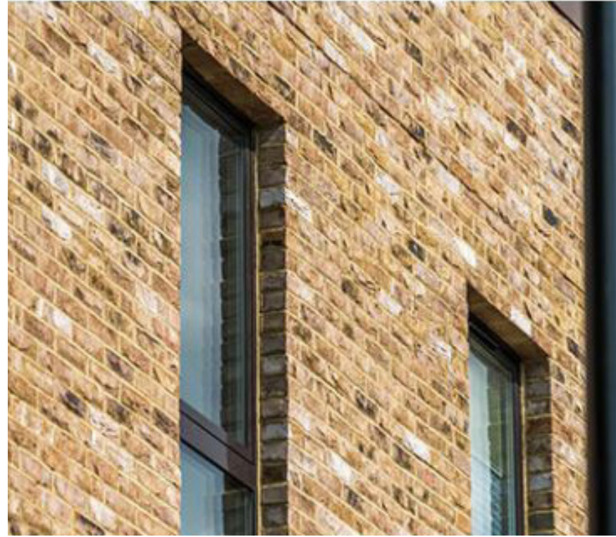
Brick slip example - Leighton Road Residential
