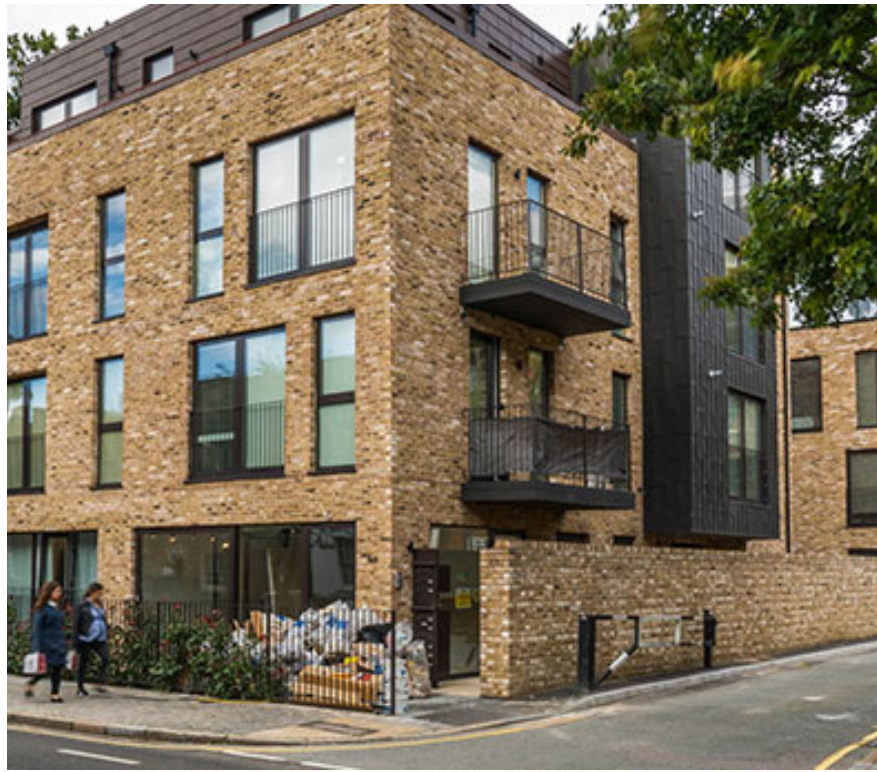
Brick slip example - Leighton Road Residential
