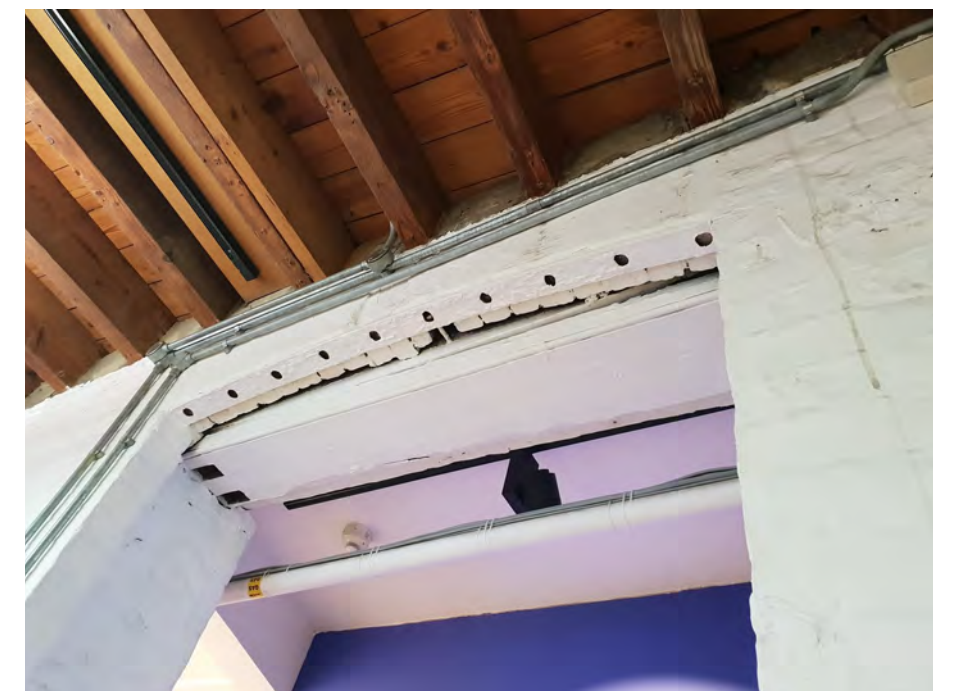
Figure 46: The Ground floor of the old Stables, the old external wall clearly highlighted with a n iron plate which formerly held bars.
