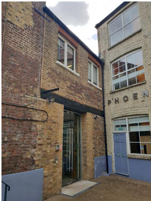
Figure 47: The façade to the extension to the rear of No. 65. This is indicated as a void space in maps from 1881, and the timber beam appears to be original.
