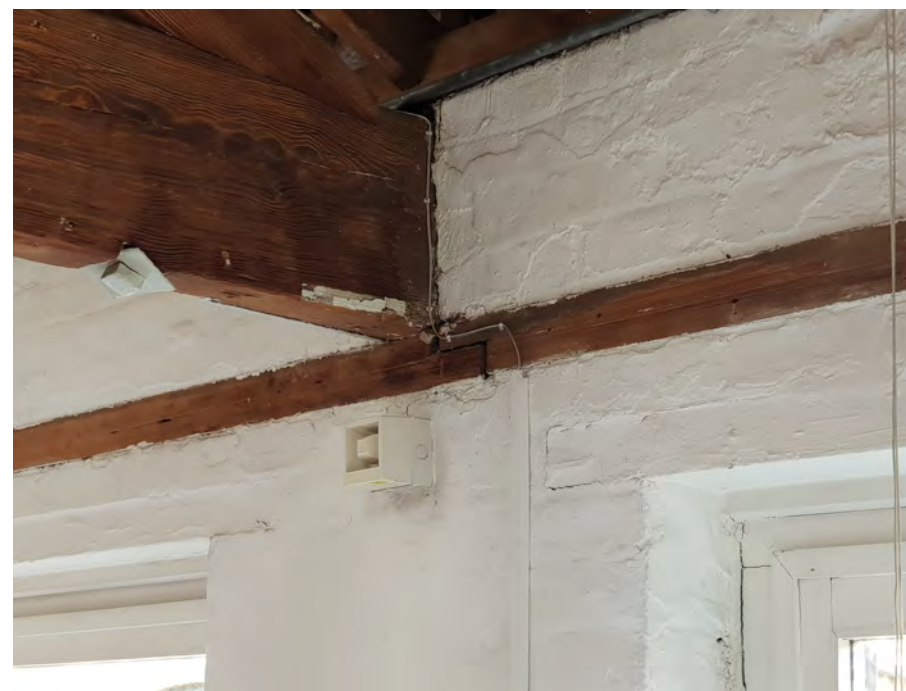
Figure 45: Trusses sitting on a timber wall plate on the second floor of the Old Stables Extension, lapped joint is clearly visible.
