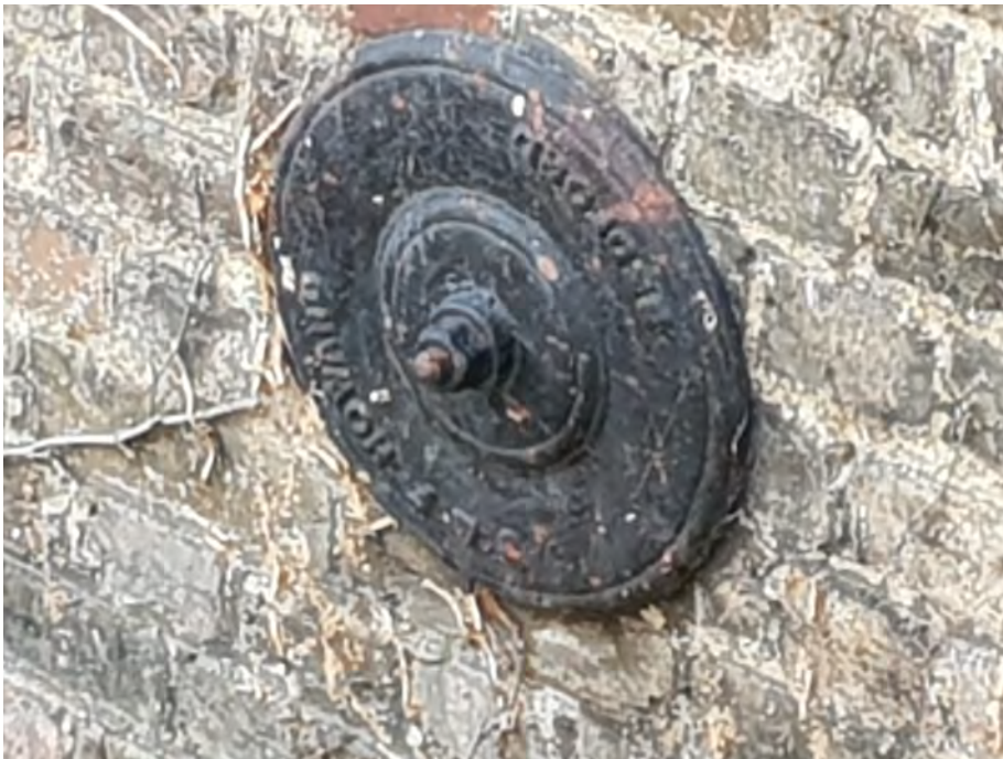
Figure 42: A Patress plate from the east façade of the extension to the Old Stables
