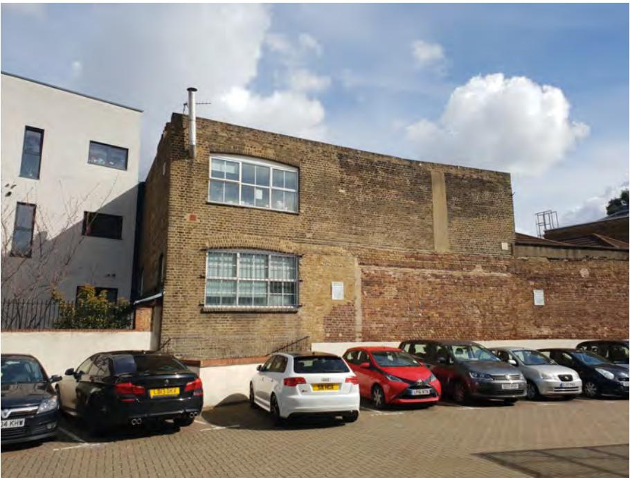
Figure 56: The rear of Nos. 67-69. the red brick appears to date from the same period as that found within No. 65, dating this to the early nineteenth century. Also found on this façade is later Victorian brick, and twentieth century patching in.
