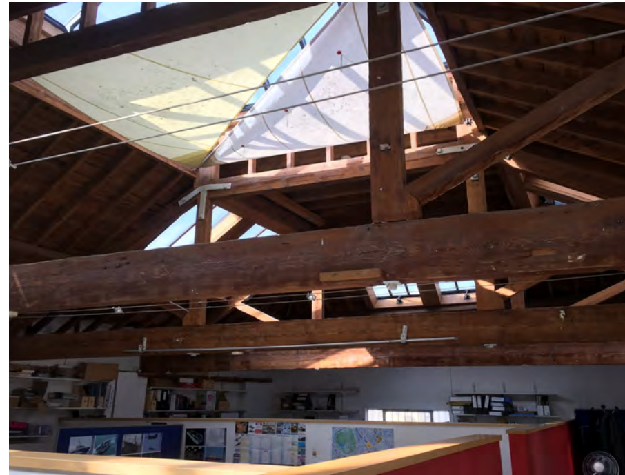
Figure 43: Nineteenth century roof structure, timber queens post trusses.
