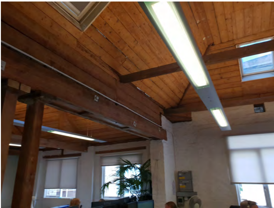
Figure 48: The roof form of the space to the rear of No. 65, also shown is the brick return which would have formed the old exterior rear wall of No. 65.
