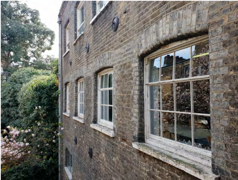
Figure 40: The façade of the extension to the old stables, glazed bricks dressing the window and older OS maps date this extension to the late nineteenth century.
