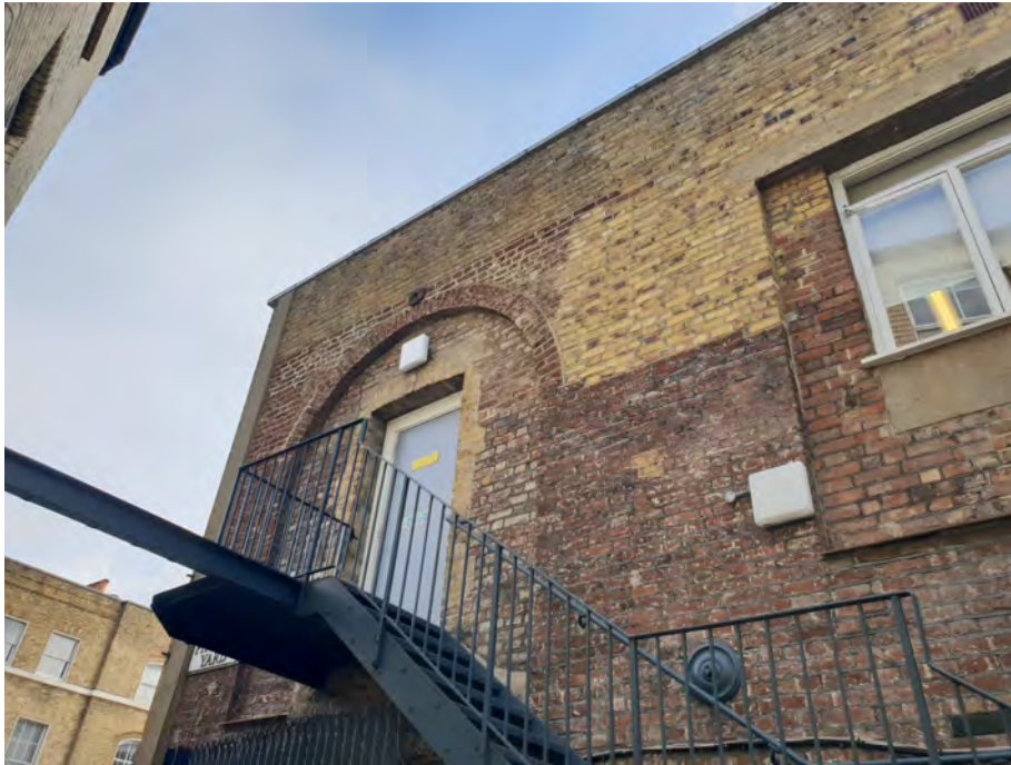
Figure 35: No 65 to the inner courtyard, showing different types of brick used from the early nineteenth century onwards.
