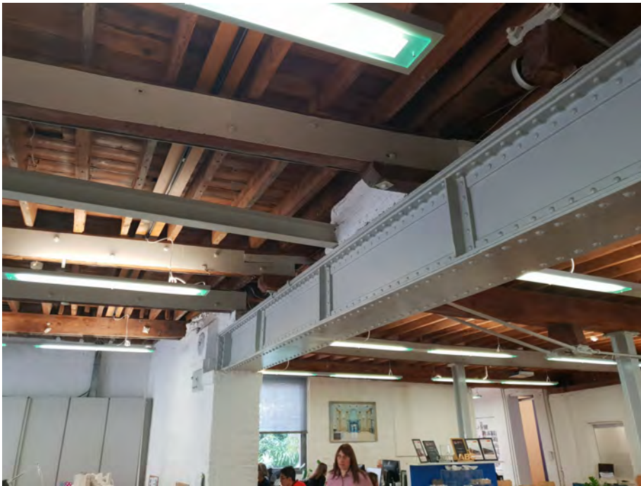
Figure 38: The large steel beam separating No. 65 from a formerly external space.
