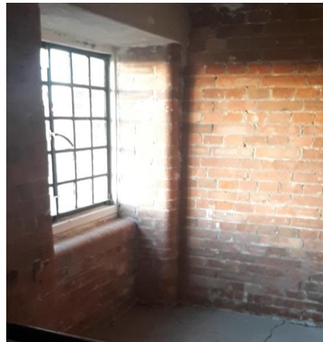
WEST-FACING WINDOWS AT EACH LEVEL
