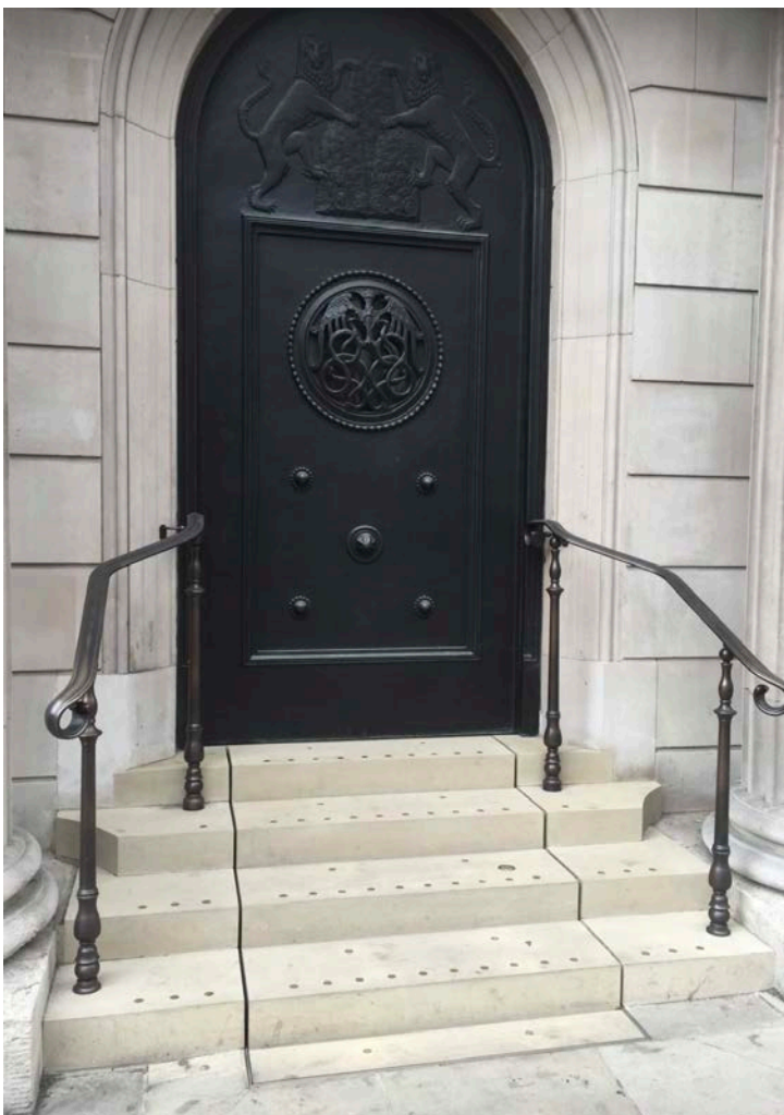
Figure 4: Sesame lift at Bank of England
