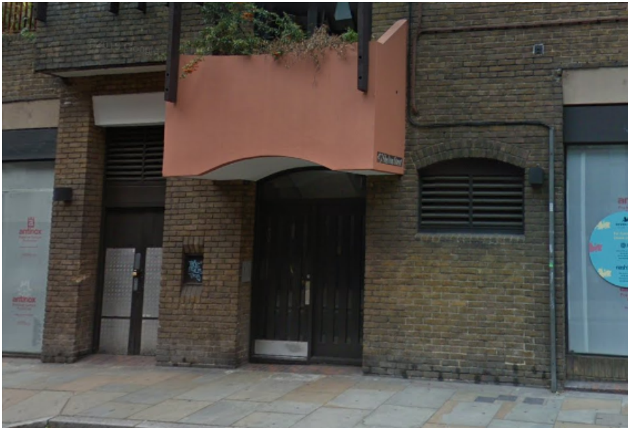
Figure 4 Existing louvres on the host building
