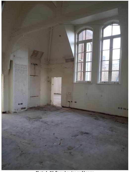
Photo 1: 4th floor showing roof beams
