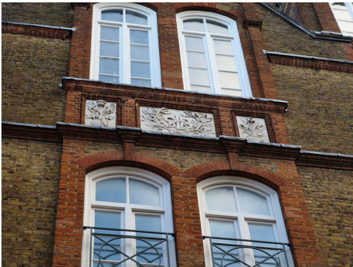
Image EDP 5: Detail of one of the relief panels with foliate decoration on the main south-western elevation.
